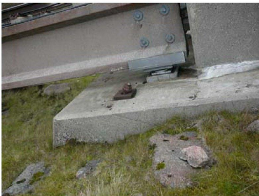
Photo [22] Typical thrust block rock anchor head.
