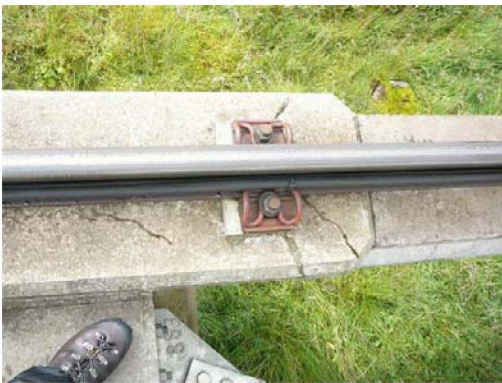
Photo [13] Pier 8 from above.
