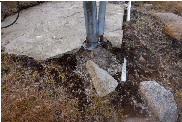
Photo 9: Upper lift base 7. Major disintegration of base.
