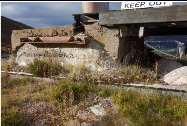
Photo 7: Lower lift top station. General disintegration.
