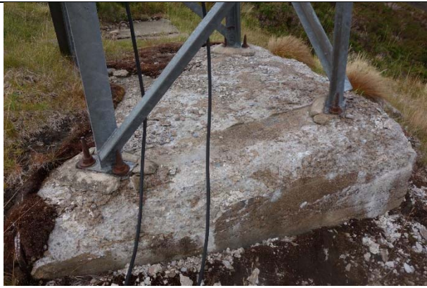
Photo 8: Upper lift base 4. General disintegration of base and bolt grout.
