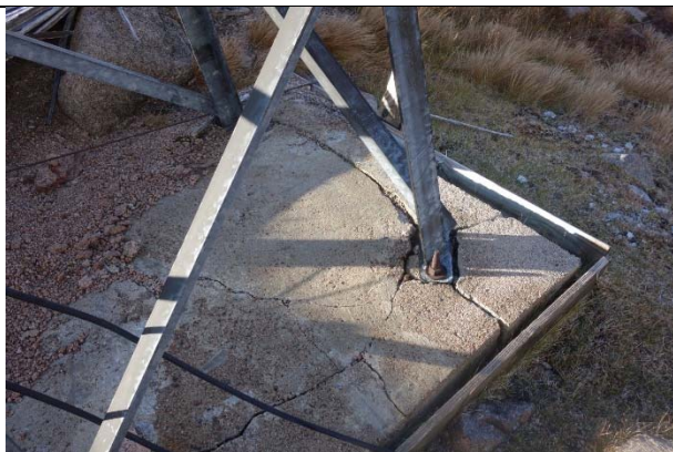
Photo 10: Upper lift base 10. Major disintegration of base.
