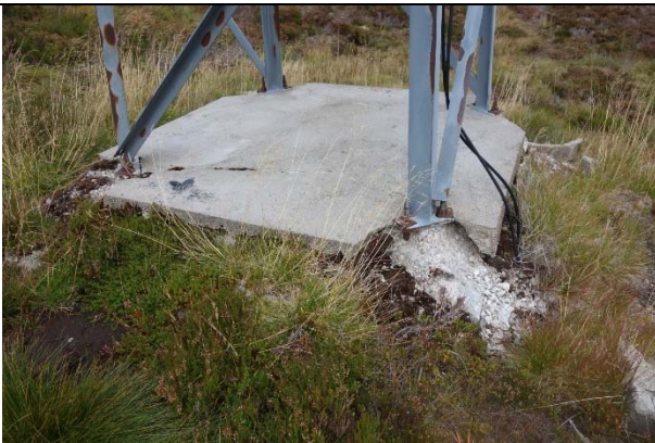
Photo 2: Lower lift base 5. Note disintegration of concrete around all bolts.
