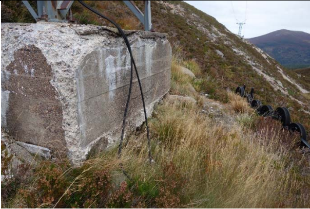
Photo 1: Lower lift base 4. Note particularly undermining of lower edge and no cover.
