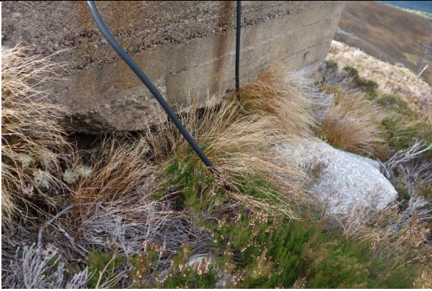
Photo 4: Lower lift base 12. Note undermining of base.
