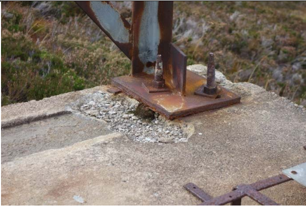
Photo 5: Lower lift base 12. Note disintegration of concrete surface around all bolts.
