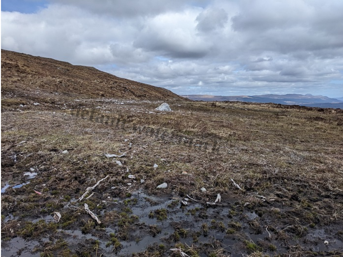
Restoration of the temporary access track, constructed around the east side of Ben Tee in 2023, for site investigations in Colre Glas
