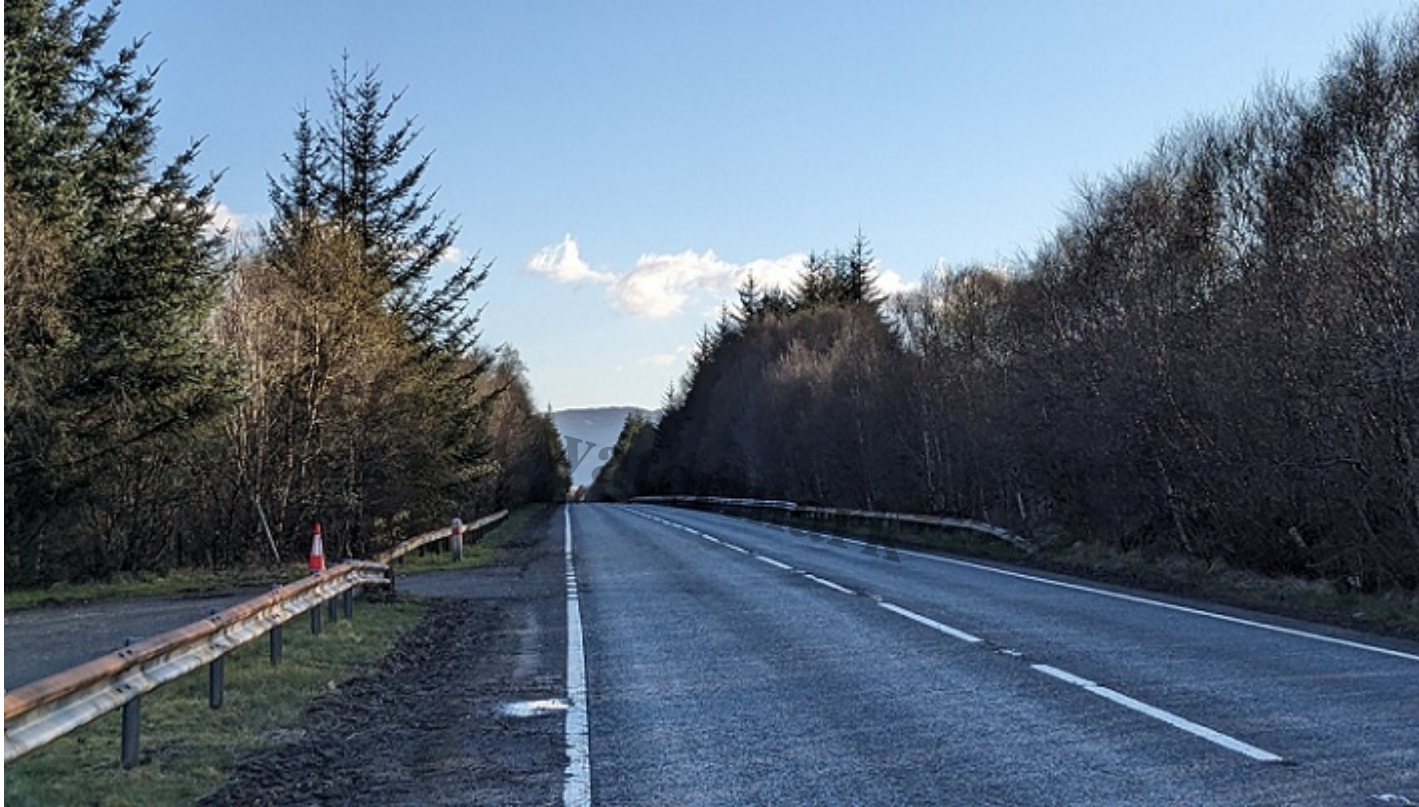
Looking West along the A82 from the large car parking area opposite Upper Glen Falcon
