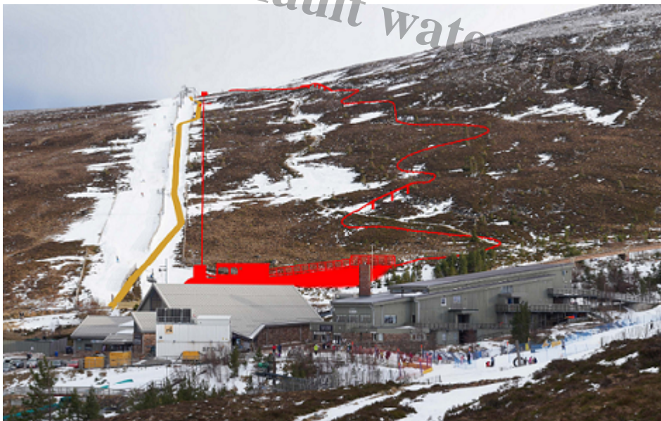
The red shows the line of the coaster and bottom station, the tan the line of the 'maintenance and emergency' track. Photo montage from LVA Graphic 5 Credit Brindley Associates
