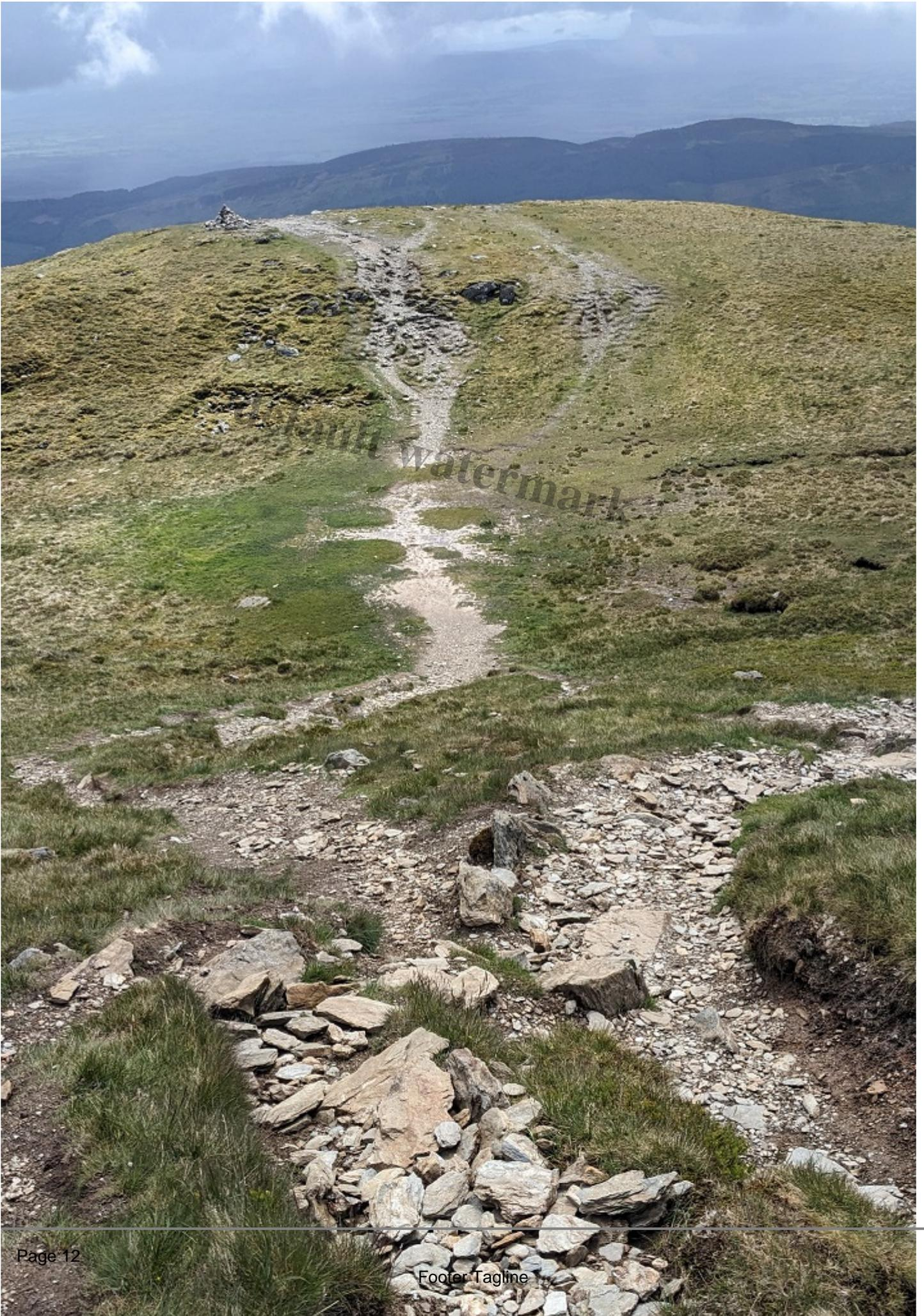
This upper section of the path had, like the lower section of path, been subject to repairs/construction work before the Mountains and the People Project and, in 2021, at the time of my last visit the remains of stone steps were still visible on this section. Without ongoing maintenance, much of the path work undertaken by the Mountains for People Project could end up looking like this.
