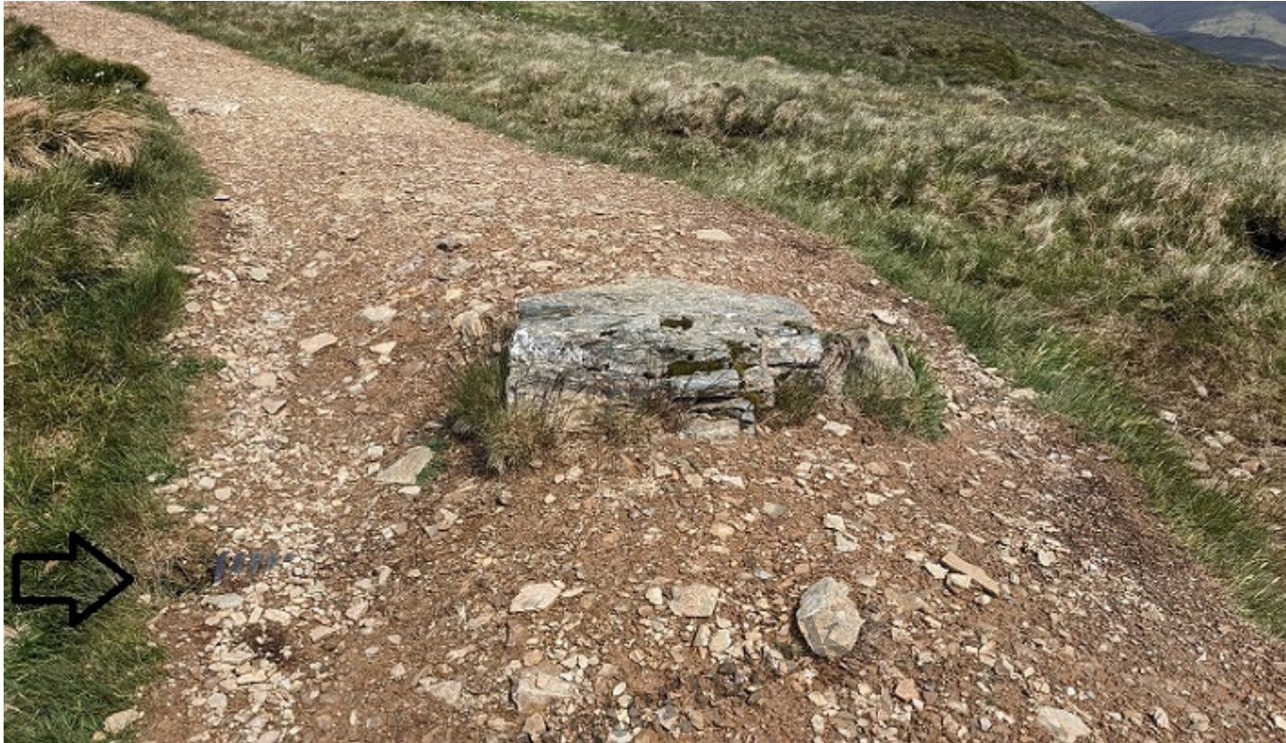
Culvert appearing by a step, stranded by erosion.
