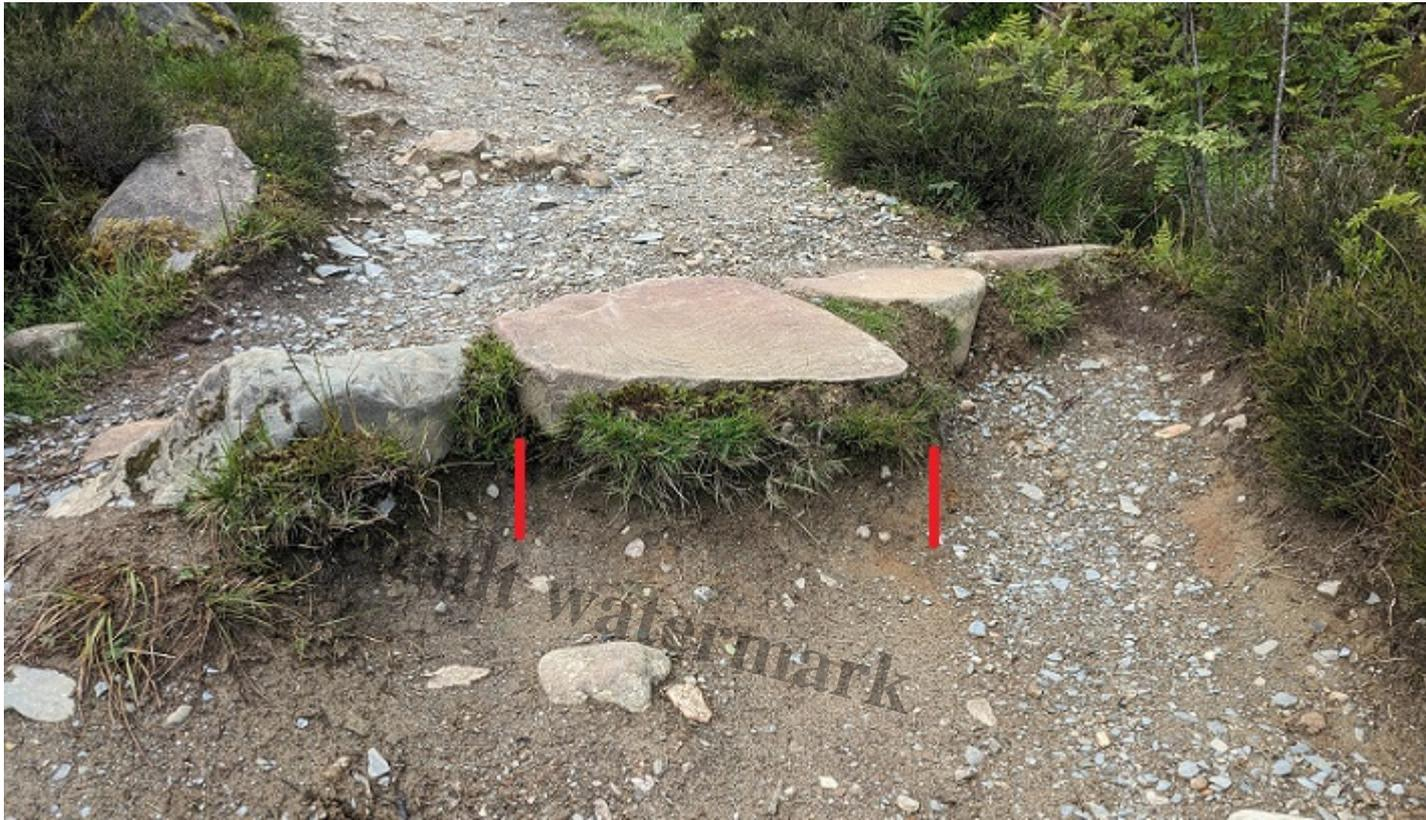
Red lines show just how much ground has eroded out below step
