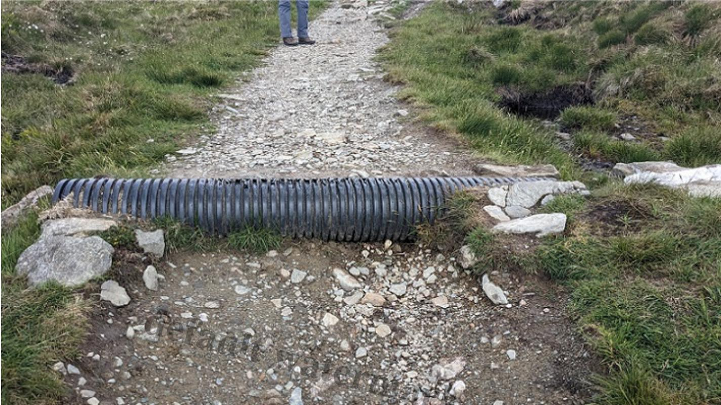
The original surface on this section of path, constructed sometime between 2016 and 2018, has completely eroded away exposing the plastic culvert which is now disintegrating
