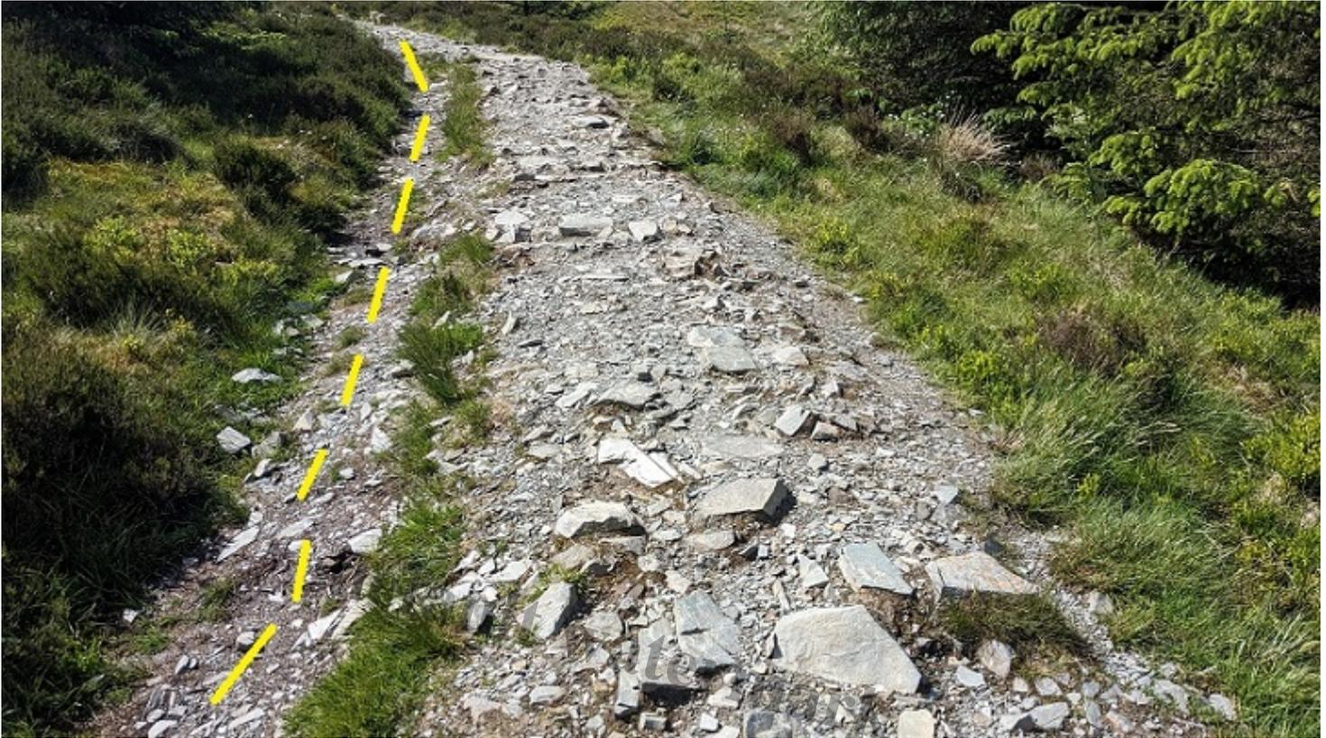
There are similar design failures on some of the flatter sections of path. Much of the fine material on this section had already washed away in 2021 (see below) leaving an uneven surface that was difficult and uncomfortable to walk on. As a result people soon started to walk along the ground between the edge of the path and what was a drainage ditch.
