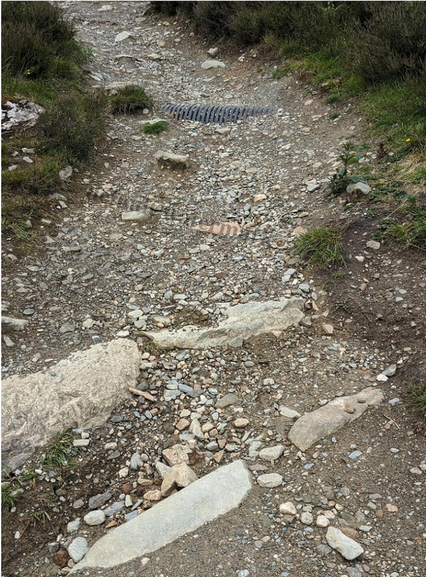
In-filled cross drain with emerging culvert behind. The material blocking the drain could be used to help cover up the plastic pipe above.
