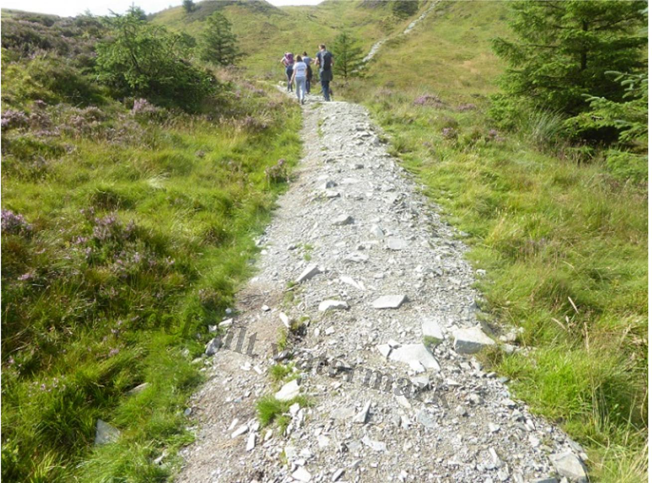
The same section of path in 2021, showing the drainage ditch on the left (already filling in with vegetation).
