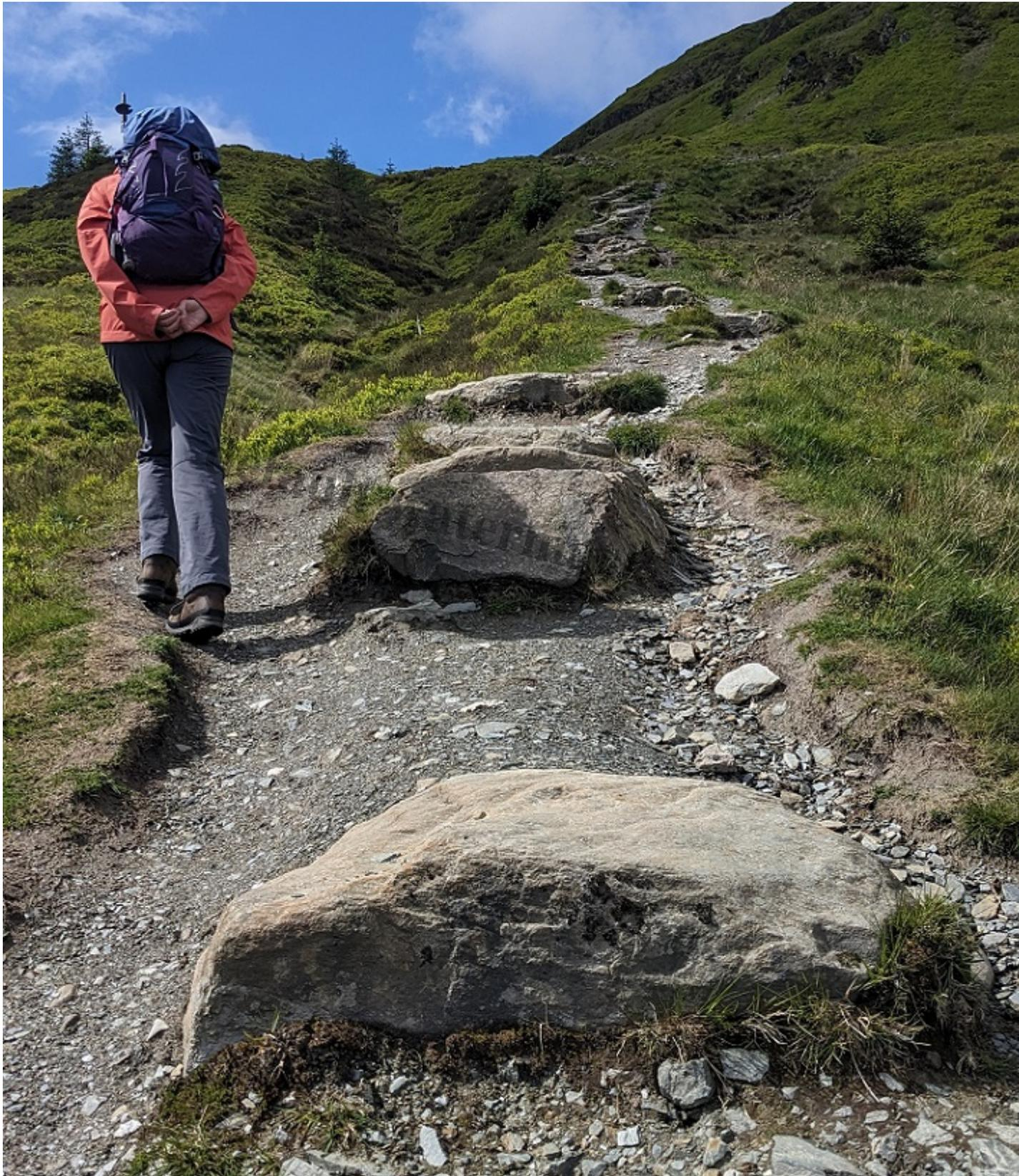
A section of path where the stone steps have become barriers- built by contractors engaged by the Mountains for People Project. Note how the right side of the path has now become a drainage channel where all the finer material has washed away.
