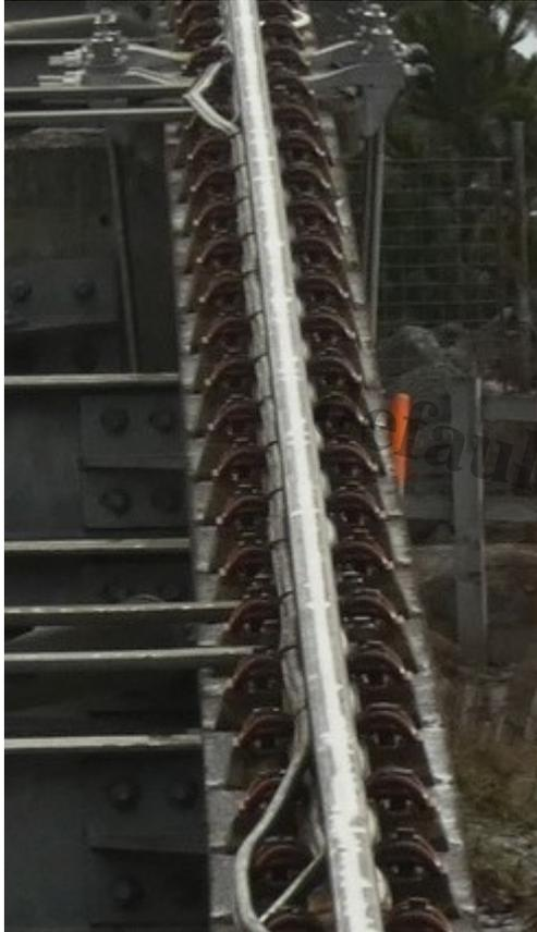
The shiny mid- section is where the bogie wheels are touching the centre of the rail with lateral shiny bits where the wheels touch now and again.
