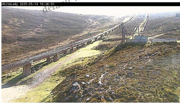
This photo, at the passing loop, better shows all the steelwork which has been added to the funicular viaduct to hold it together. Note the figure working on the structure. Photo courtesy CM(S)L webcam.
