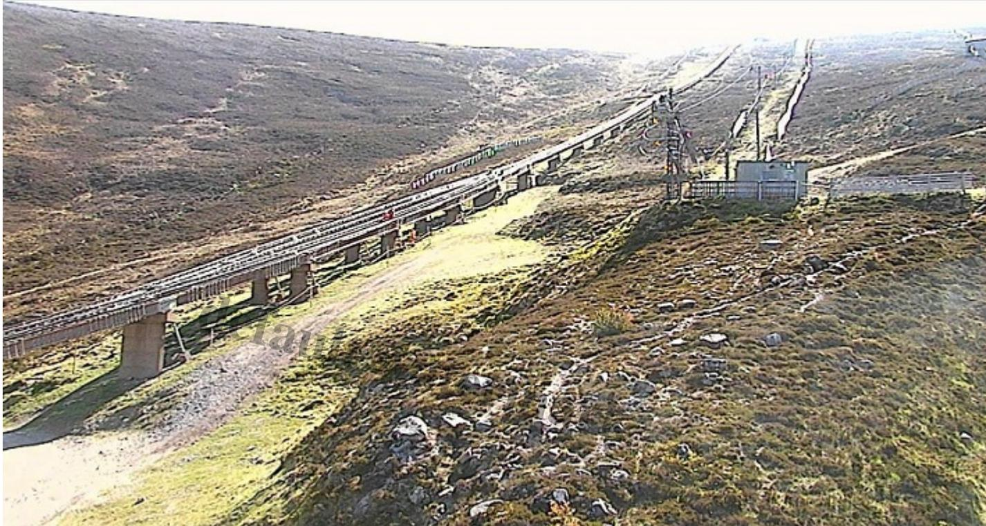
This photo, at the passing loop, better shows all the steelwork which has been added to the funicular viaduct to hold it together. Note the figure working on the structure. Photo courtesy CM(S)L webcam.
