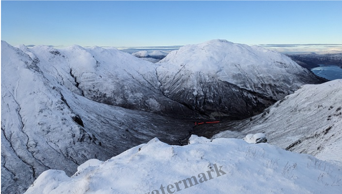
The location of the proposed mast and track from near the summit of Biod an Fhithich, the Corbett Sgurr Mhic Barraich right of centre and Skye beyond
