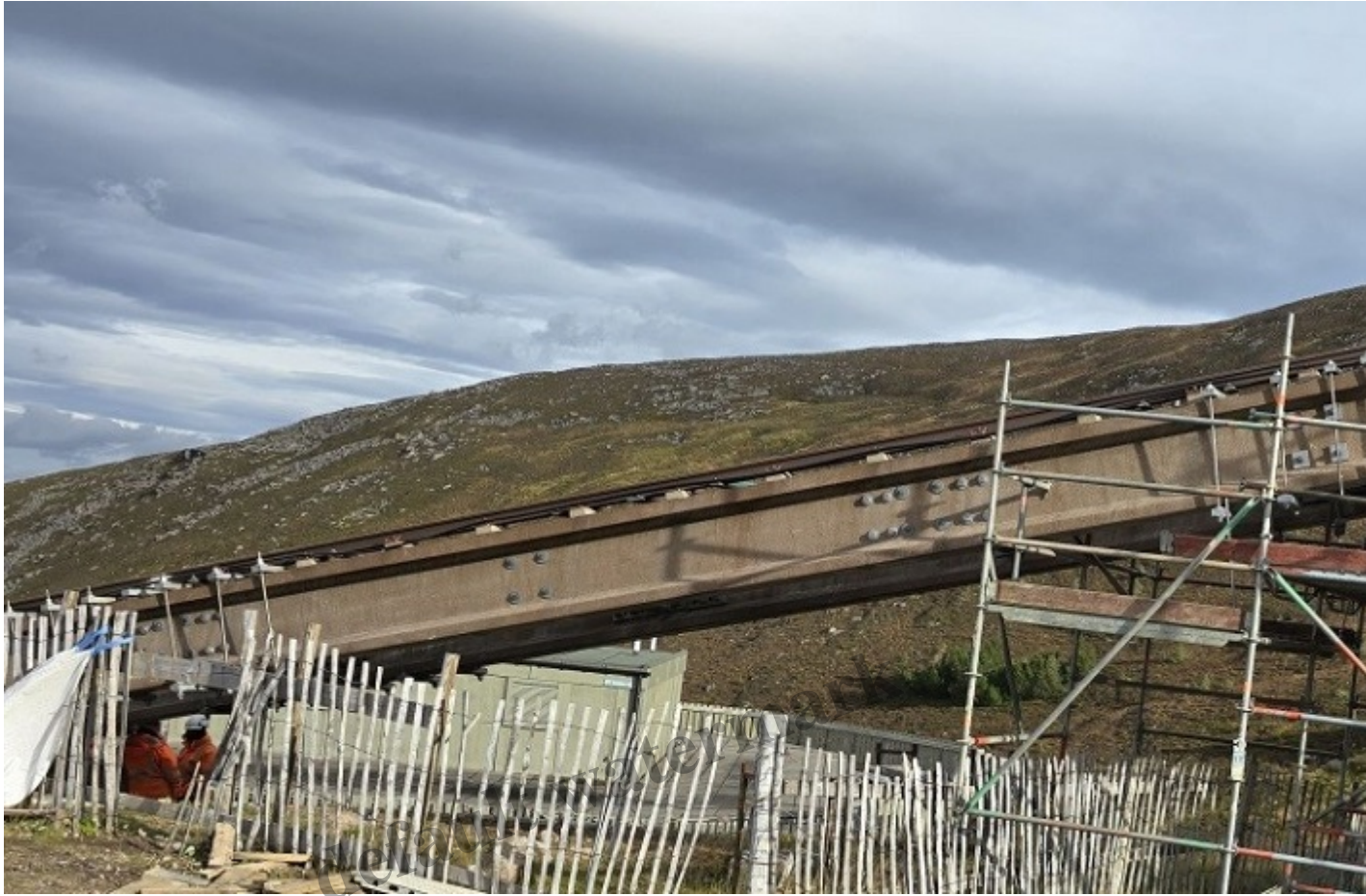
Workers by pier 50/51 on left of photo. 4/10/24.
