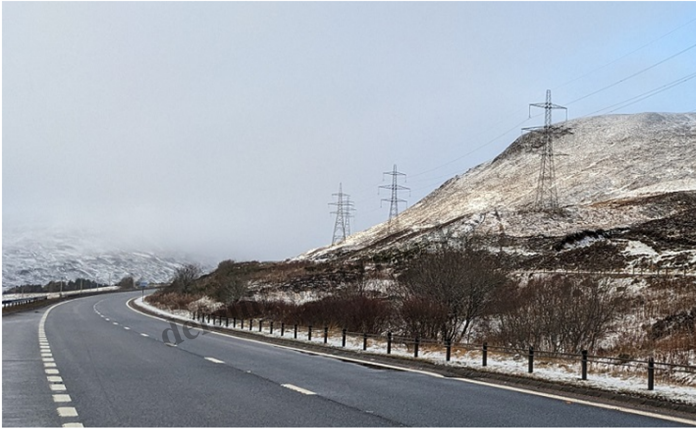
A section of the A9 central reservation approaching Dalnardocho viewed from a layby on the northbound carriageway 4th January
