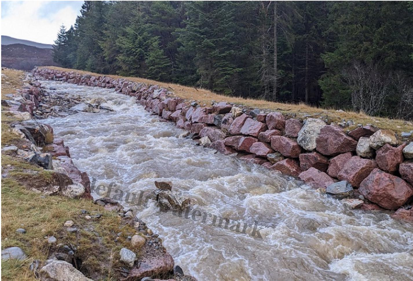
Stranded rock on boulder in foreground with differential erosion of the base of the channel evident from the "dry" area behind.
