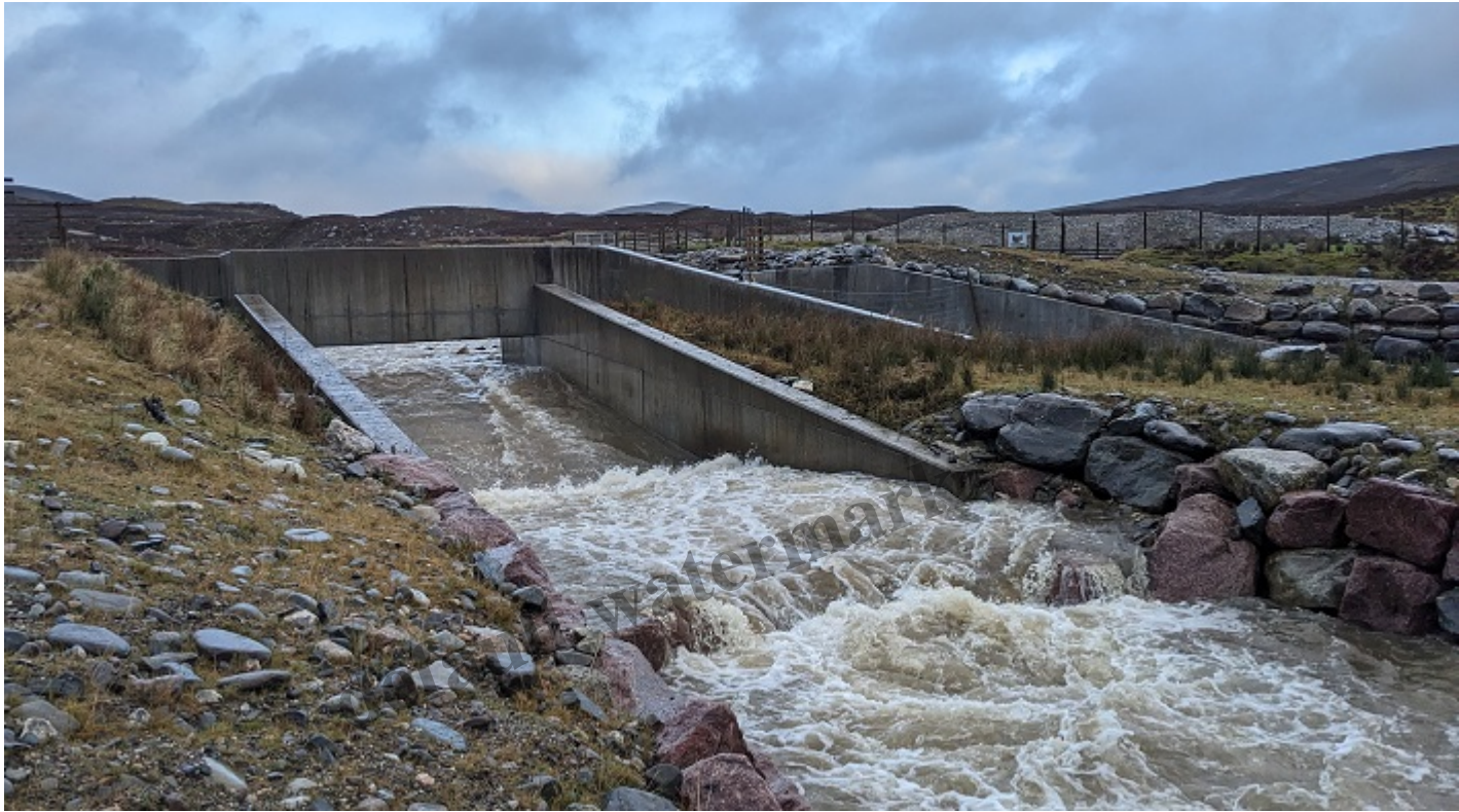
The intake to the Gynack overflow from below 31st Dec 2024
