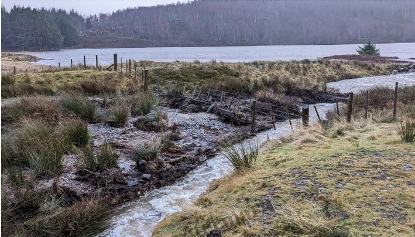
The outflow of the overflow channel viewed from the eroding section of bank. Note the difference between the still half bare bank in the foreground with the heavily vegetated bank beyond
