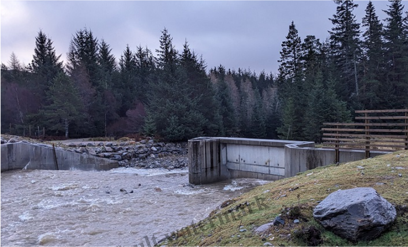
The intake to the Gynack overflow from below. 31st Dec 2024
