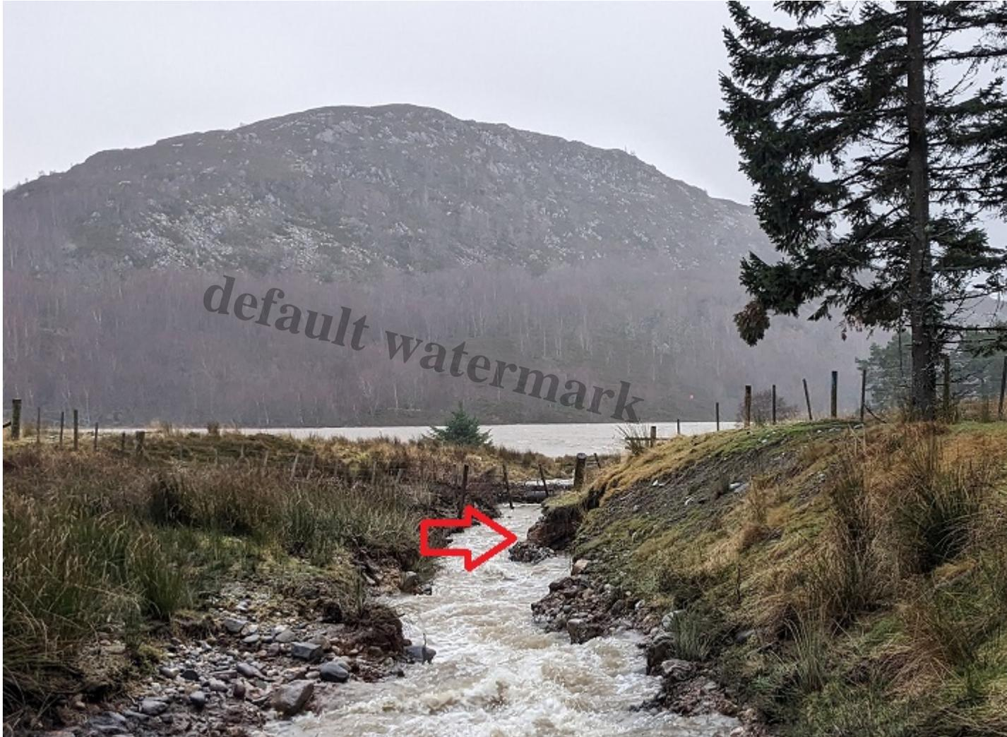
The lowest section of the channel is surprising narrow (and deep) and looks certain to sweep away a further section of the embankment on the right.
