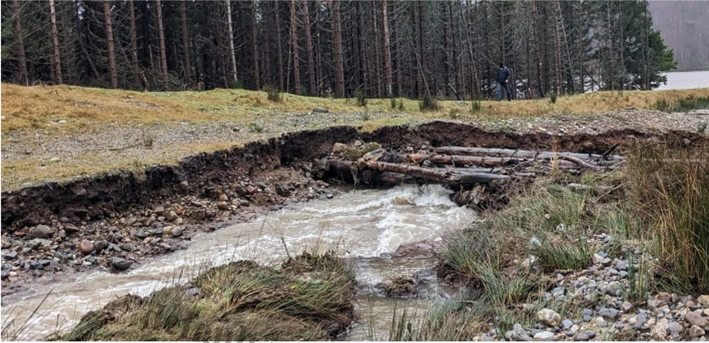
Near the bottom of the channel, with Loch Gynack visible behind. Note how the bank at this point has been built constructed with shingle, washed down by the previous overflow channel, not earth.
