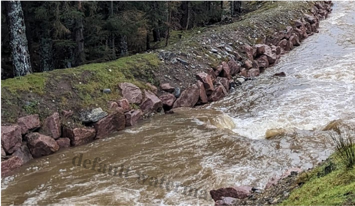
Note how the earth heaped on top of the rip rap bouldering has been eroding just to the right of the tree and along the bare area which starts by the bottom step
