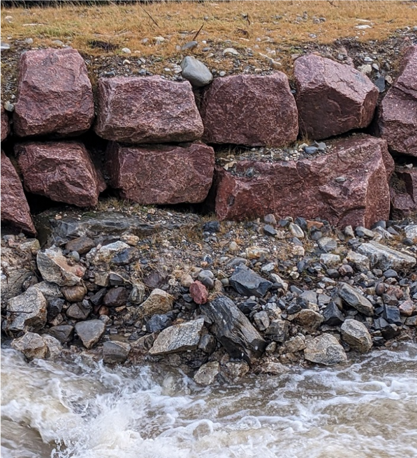
A section of rip rap bouldering that has now been partially buried
