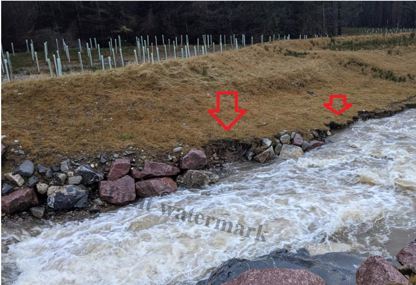
The gap in the protection was probably filled with two or more smaller boulders. Note how the gently sloping earth embankment downstream has started to erode.
