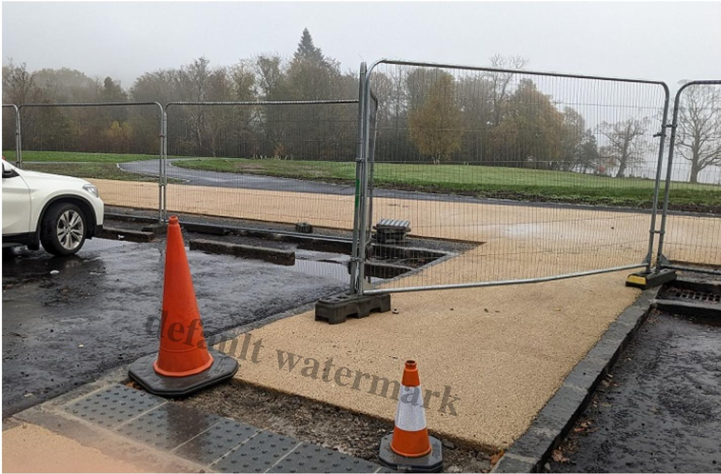
An unfinished section of coloured asphalt path crossing the car park one of dozens of bits of snagging work that remained to be completed on 28th October. The black path behind is due at a later date to be upgraded to coloured asphalt.
