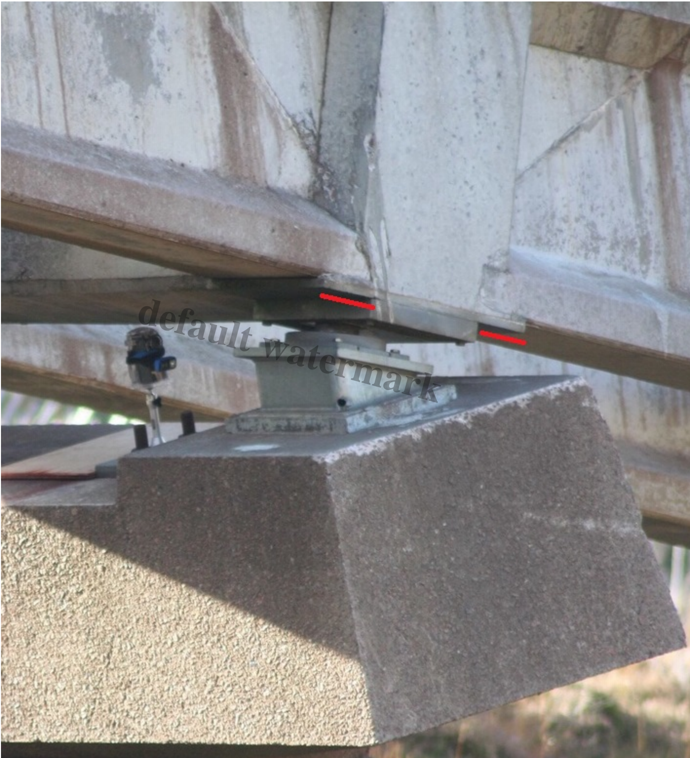
The plate supporting the end of the beams
