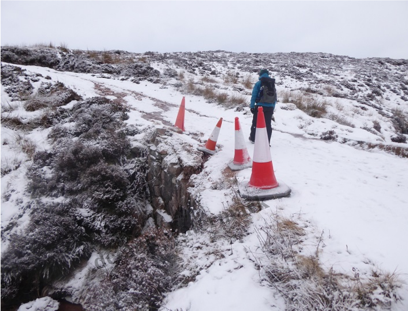
The damaged bridge last New Year
