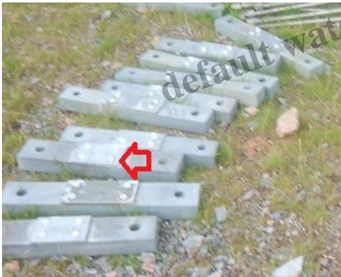
There are four blobs of grout on each plate
