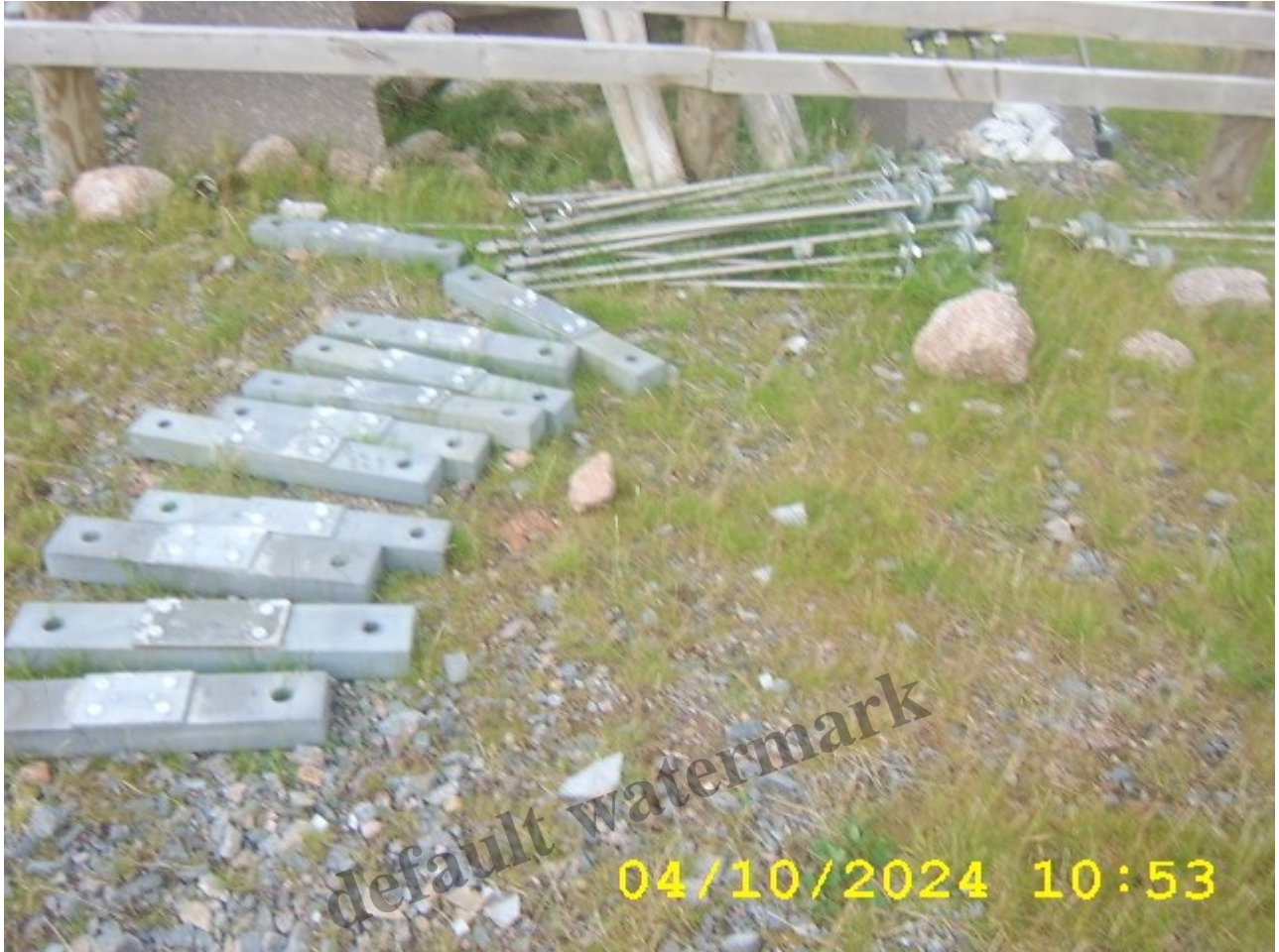
Photo. Type 1 brackets off the top pier of the passing loop.
