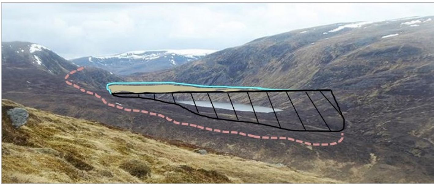
Loch a' Bhealaich Leamhain, with the dam and raised shoreline (with daily drawdown zone in brown), and the permanent access track (photo from below Carn Dearg by Nick Kempe)
