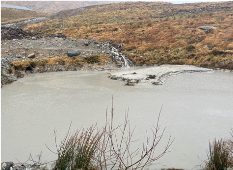
Upper Pond #2 – Small silt island remains from recent cleaning wic 12th February 2024; this is stable and sufficient capacity to receive drainage from Stack 2
