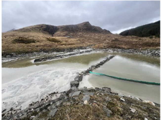
Settlement Pond April 2024 (post clearout)
