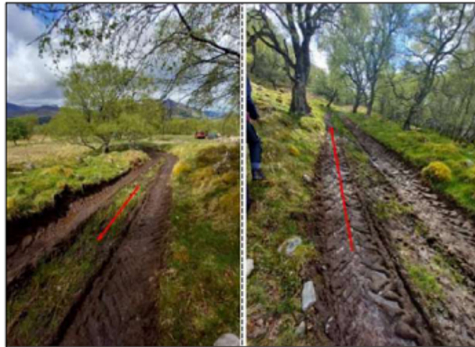
Figure 6: Photographs illustrating the condition of the access track to Discounted Option 1.
