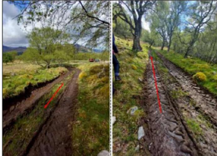
**Figure 6: Photographs illustrating the condition of the access track to Discounted Option 1.**
