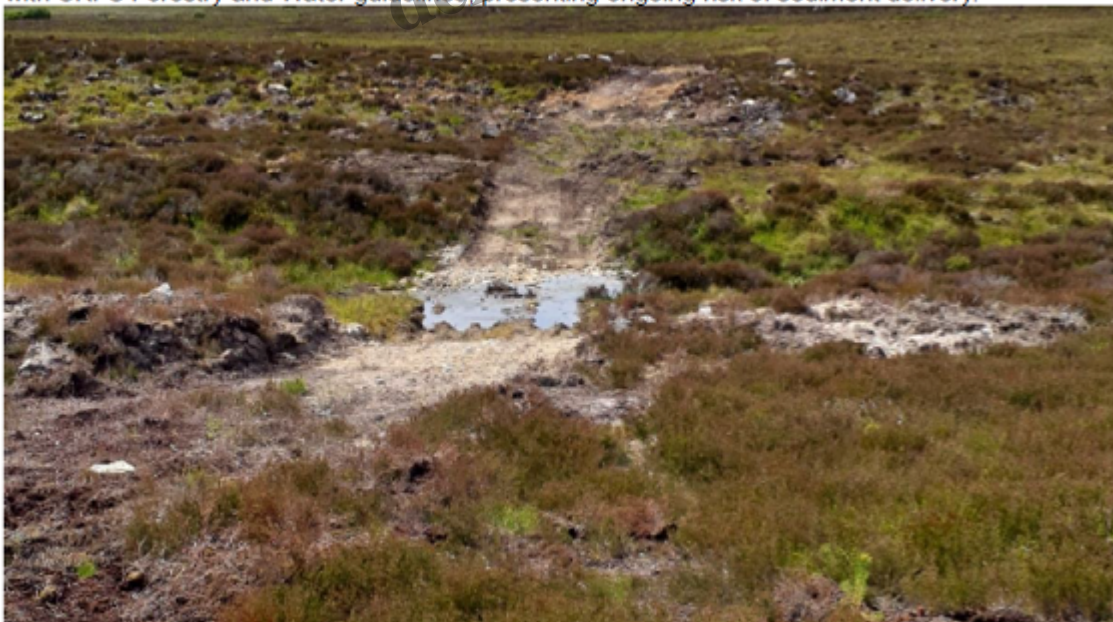
NH 9503 2819 view W Construction of new ford across Rychraggan Burn, non compliant with UKFS Forestry and Water guidelines, presenting ongoing risk of sediment delivery.
