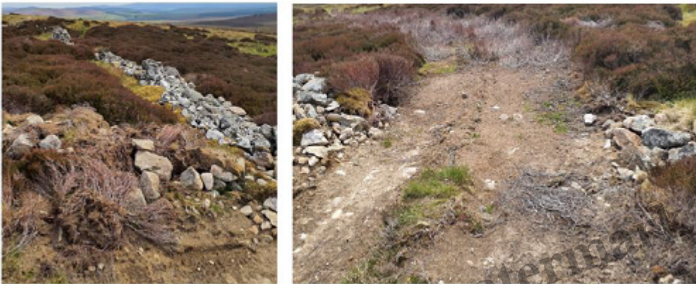
NH 9521 2875 view S Construction through a dyke that forms part of a larger enclosure.
