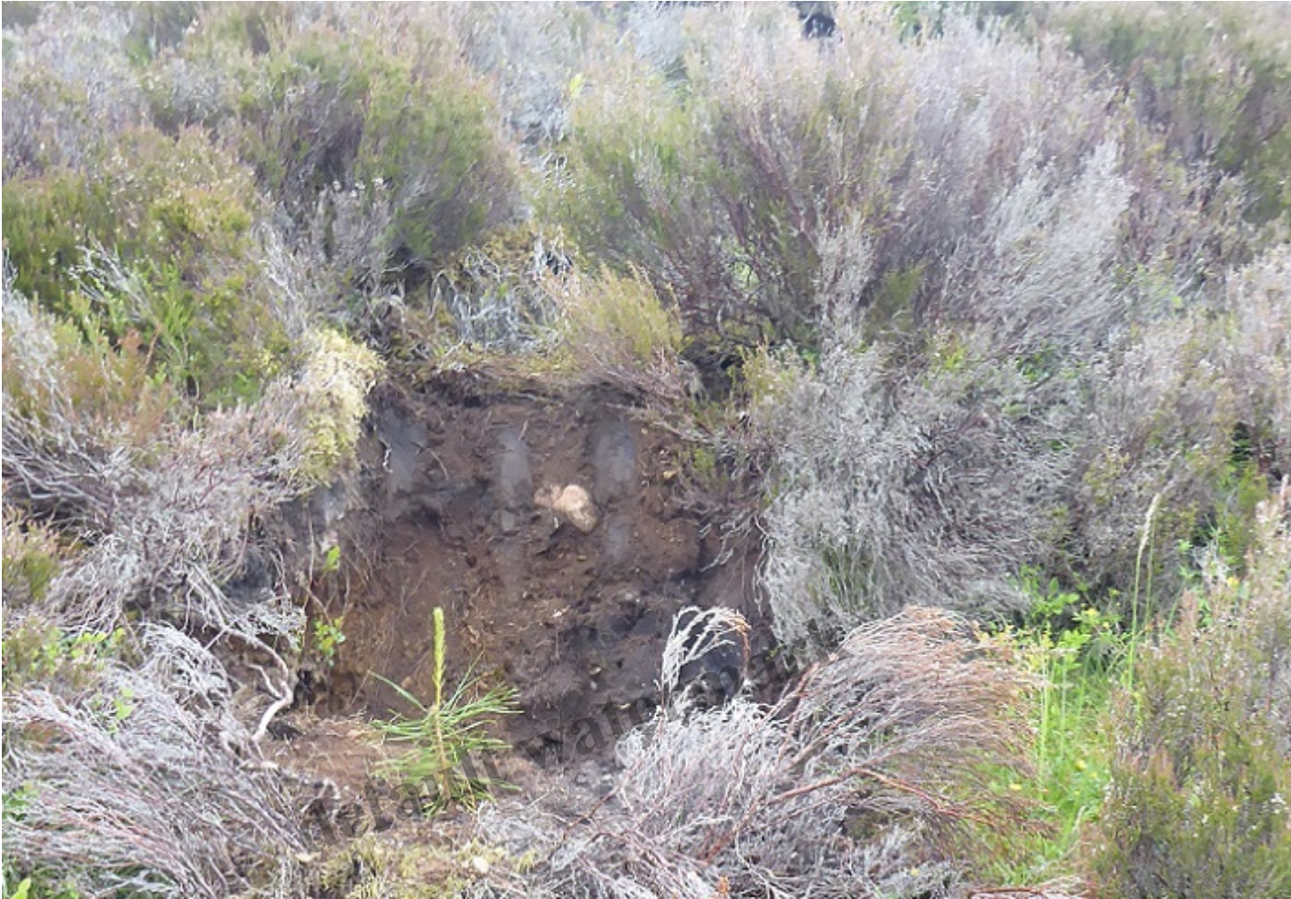
Ground excavated and vegetation destroyed to plant Scots Pine
