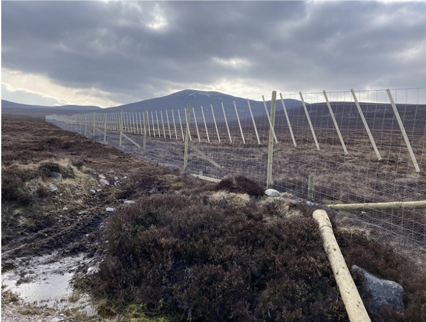
Part of three large fenced enclosures erected to create BrewDog's Lost Forest on Kinrara estate. Photo credit Dave Morris.
