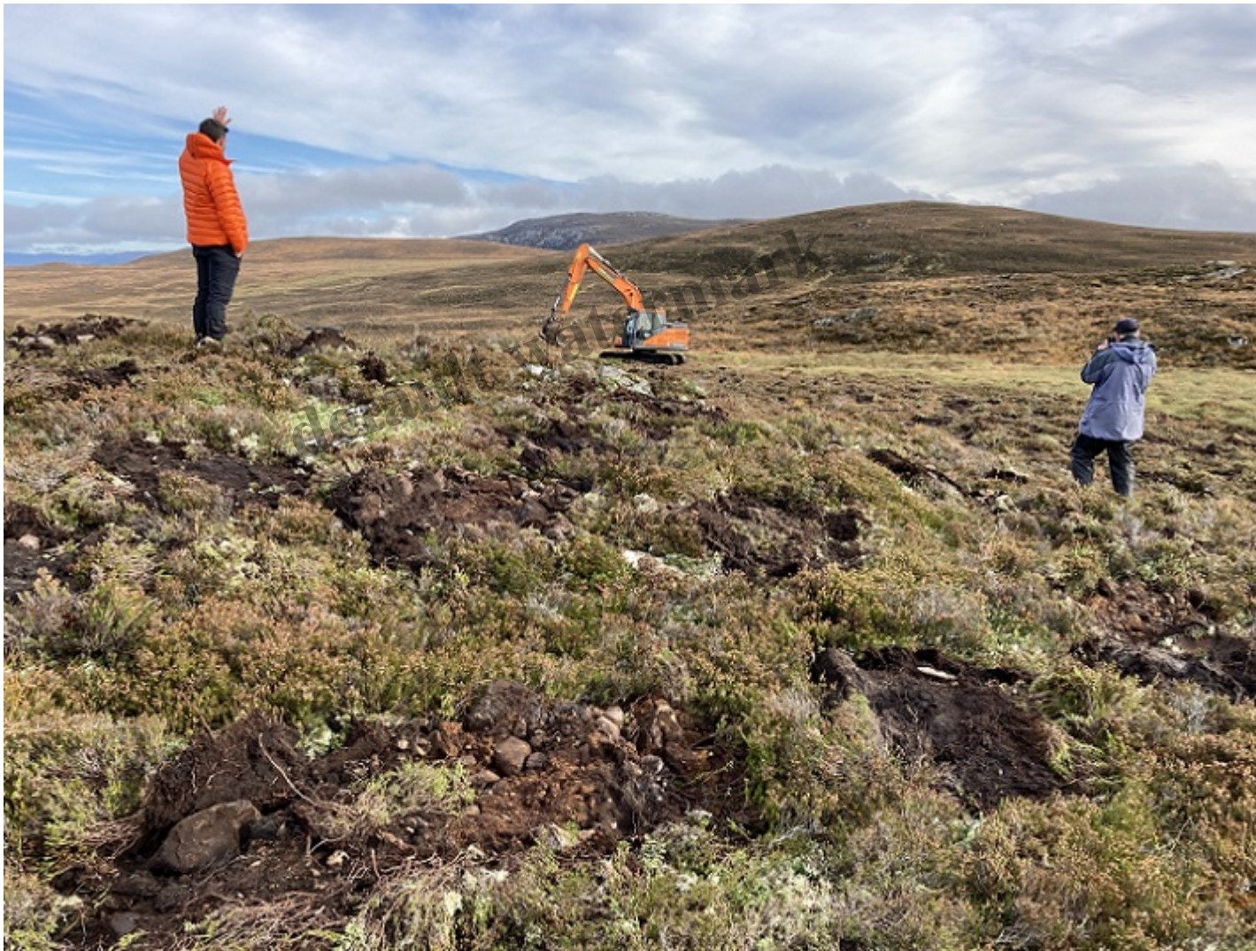
Mounding of peaty soils on abrdn's Far Ralia Estate prior to planting. Photo credit Dave Morris
