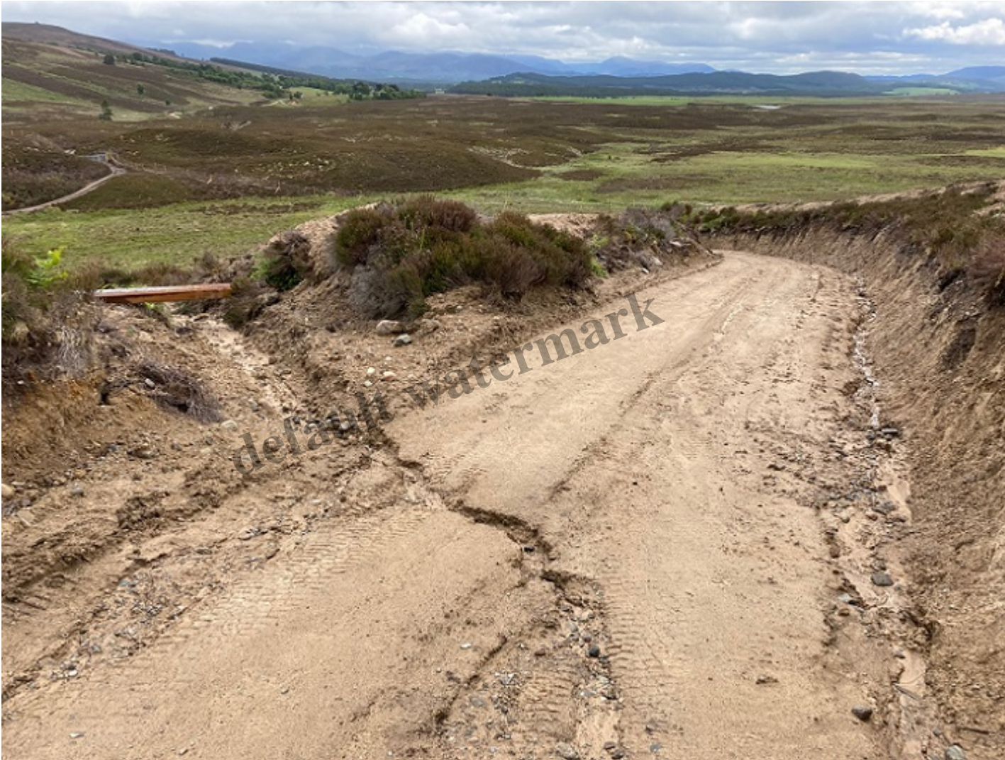
Hill road construction on Muckrach Estate. Photo credit Dave Morris
