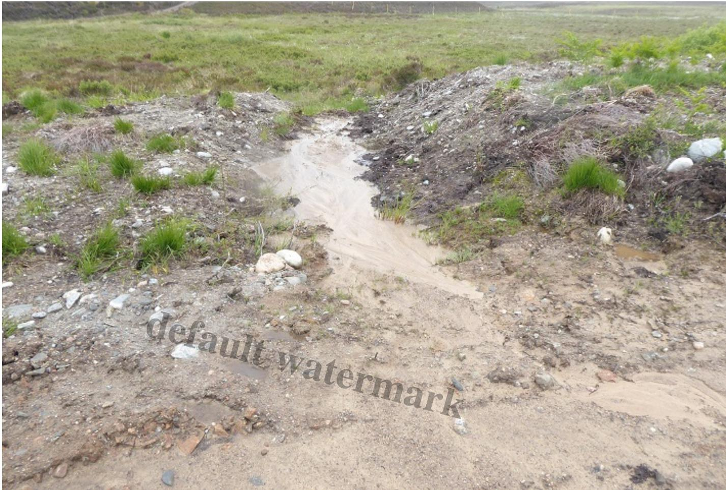
Silt washed out from the lowest drainage channel to the edge of the bog
