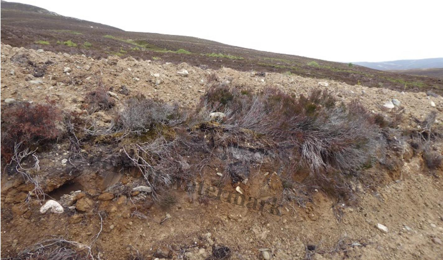
The material excavated to create the road has been dumped on either side, leaving a narrow fringe of vegetation along both sides.
