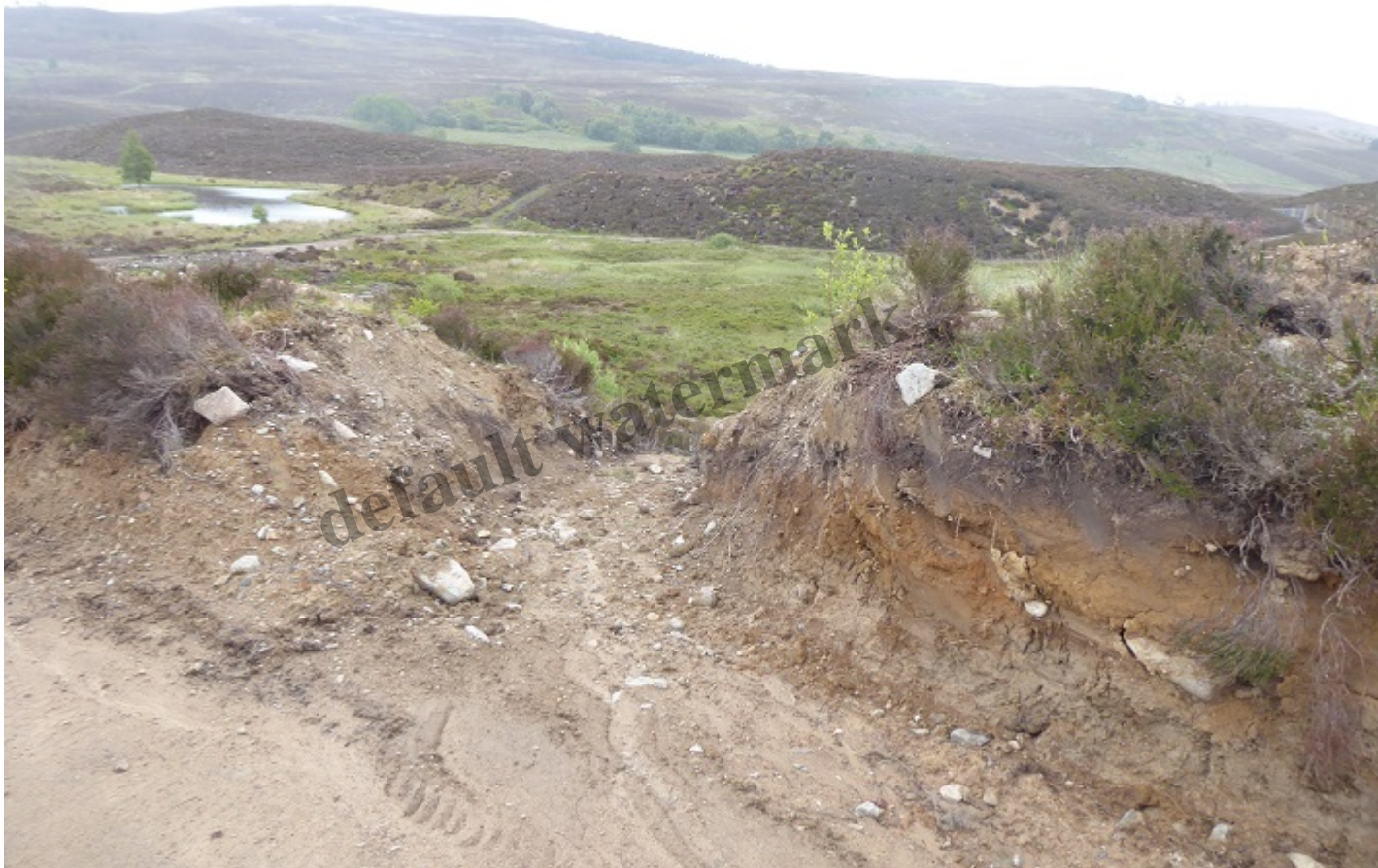
Another drainage channel looking out over the former duck shooting pond
