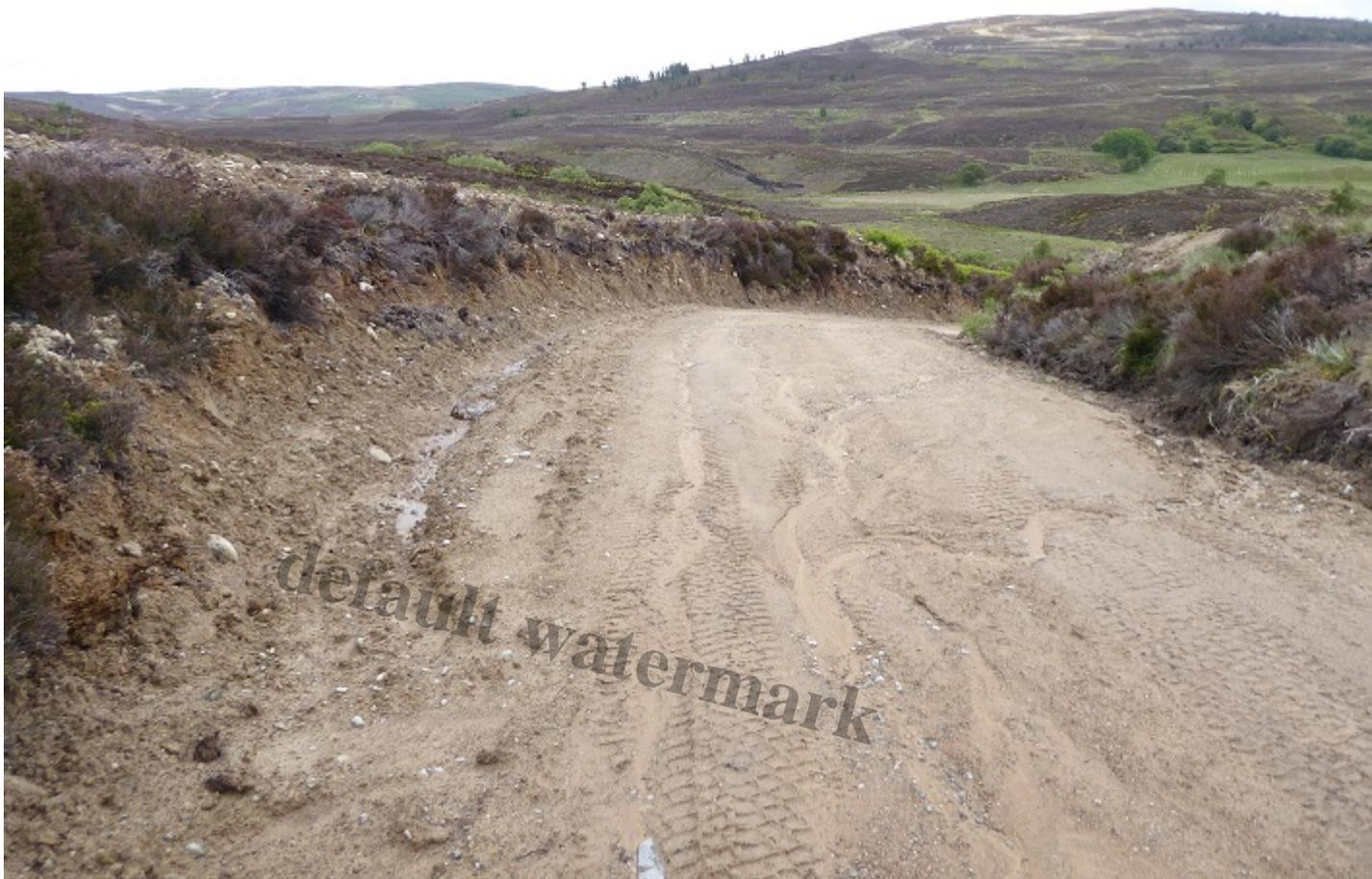
Upper section of new road, which was dug through sandy sediments originating from glaciers. Those sediments are now being rapidly eroded by water with several erosion channels visible in the photo.
