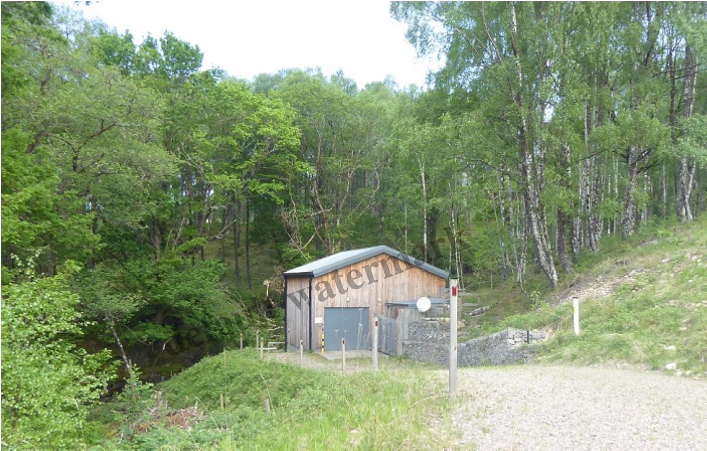
The powerhouse on the Allt Mhuic butterfly reserve on the north side of Loch Arkaig – note the wooden posts marking the edge of the new track and the plastic post on the right
