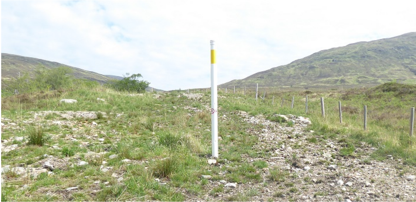
View up the pipeline from the boundary of the Allt Mhuic reserve
