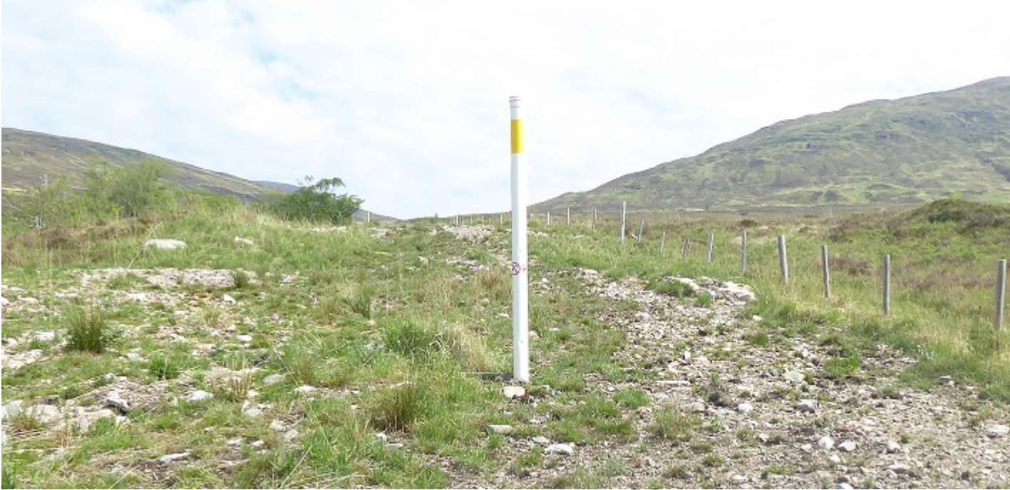
View up the pipeline from the boundary of the Allt Mhuic reserve
