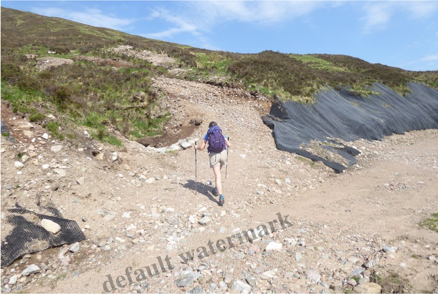
An extension of the road up onto the moorland just before the hydro intake with the plastic matting that had covered this part of the slope moved to one side
