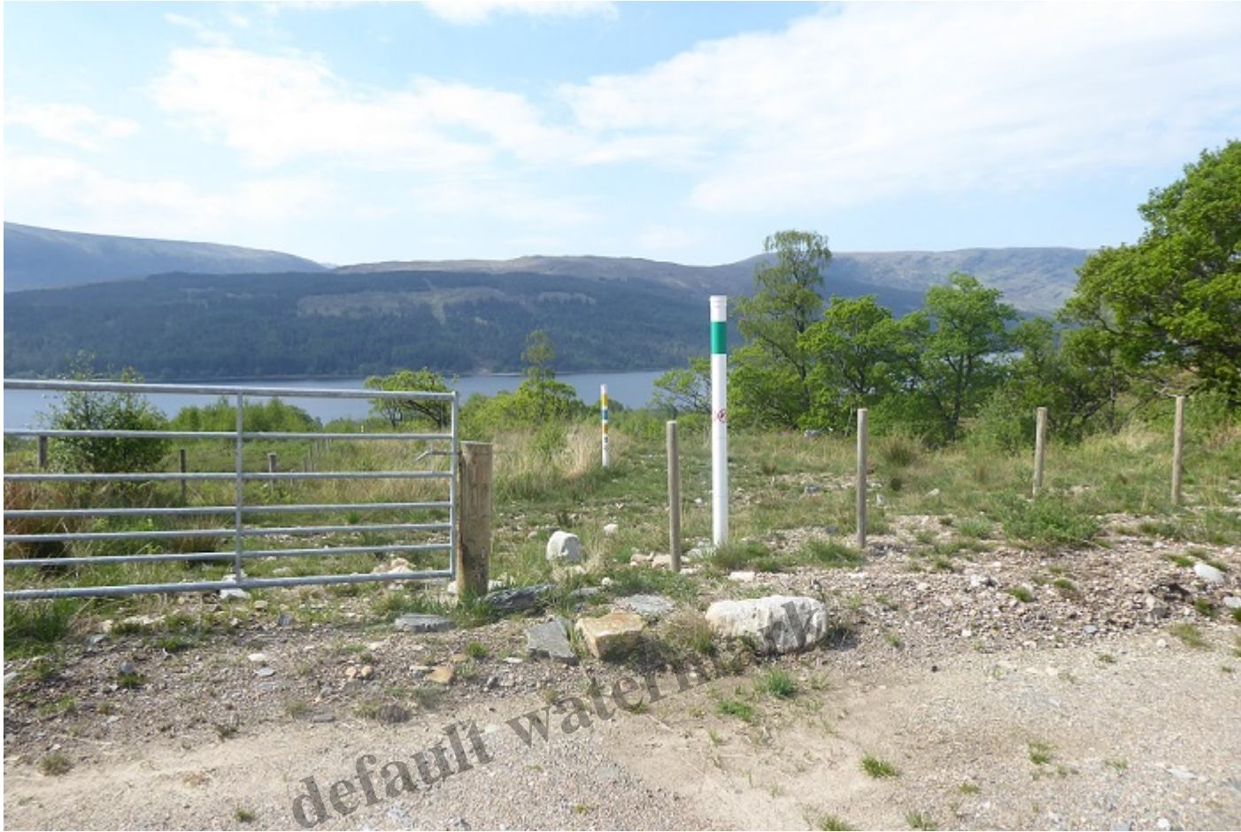
View down the line of posts marking the high pressure pipeline from the top of the Allt Mhuic Reserve
