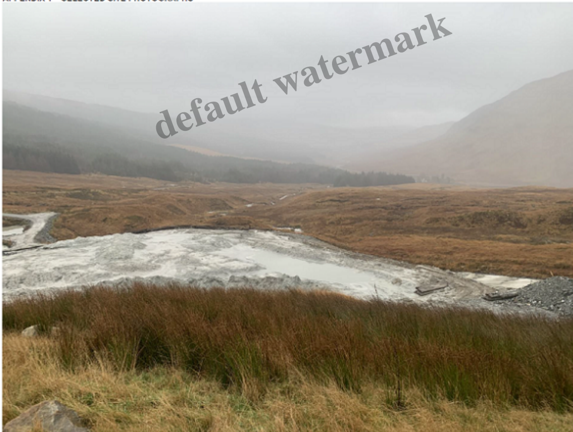
Stack 2 status 08.12.23 – Stack viewed from above. Further works are required to the surface during care and maintenance, comprising blading off and covering areas that are not used for placing tailings from pond maintenance, with geotextile.
