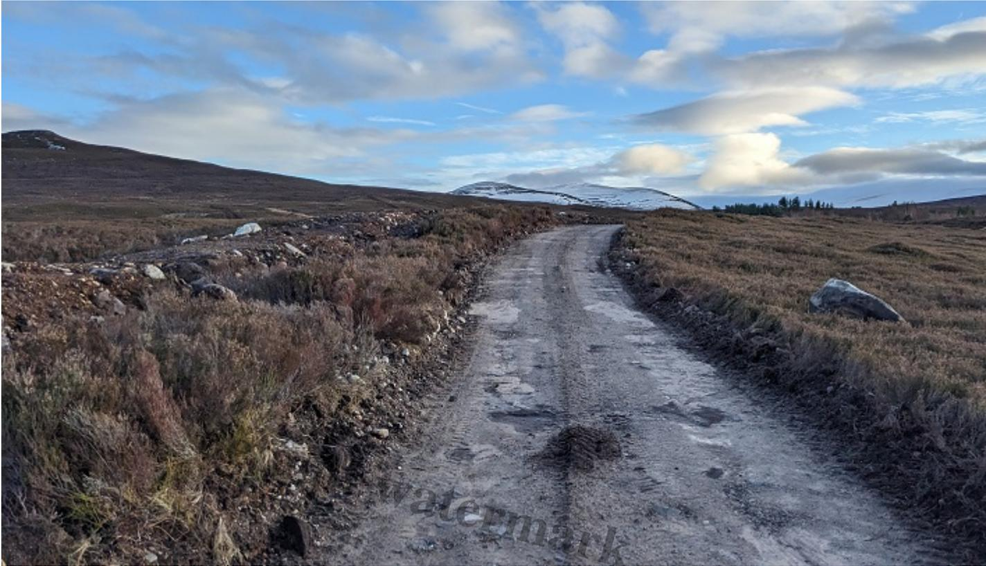
Widening and resurfacing of new road – note the new unrestored bank of soil and boulders on the left and the disappearance of the vegetated strip down the middle of the road. Photo 2nd January 2024
