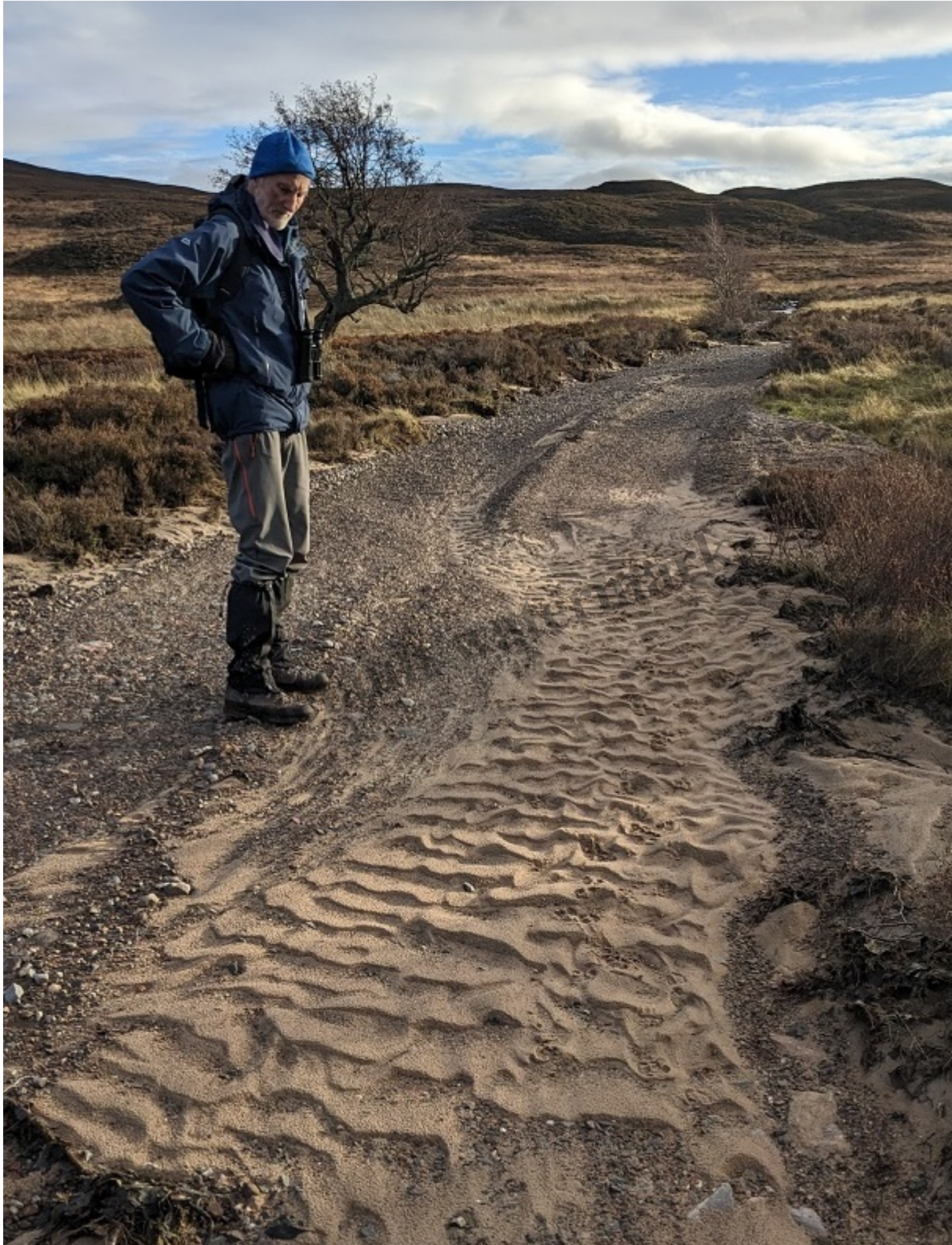
Dave Morris surveying the damage to the road by the Allt Ghuibhais
