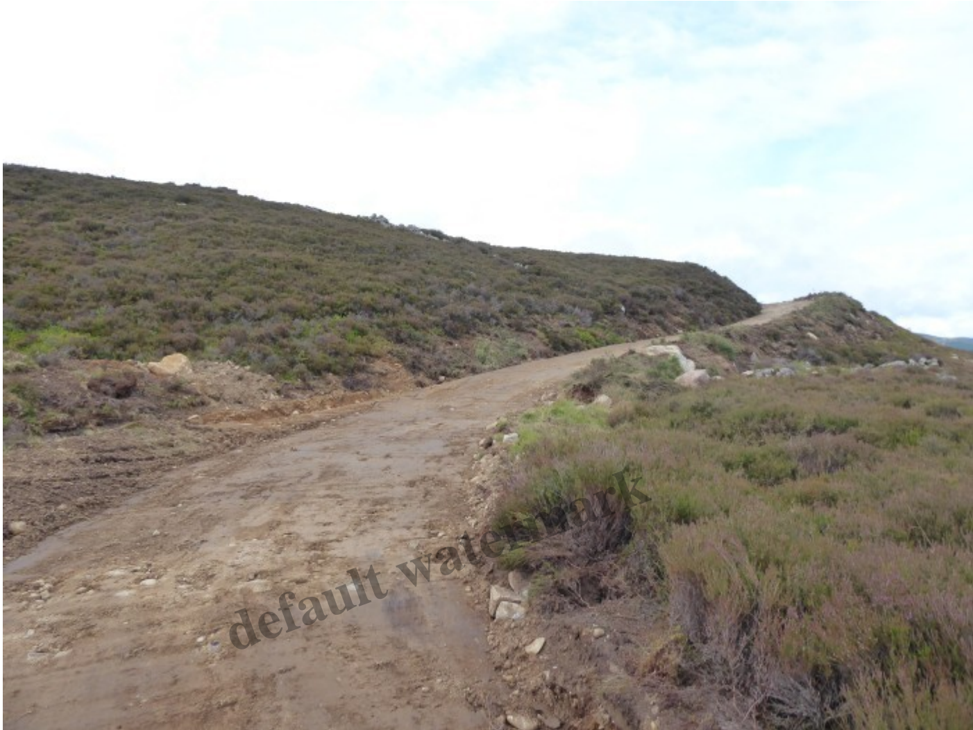
Section of road on Far Ralia as it rises over the hill before the Allt Ghuibhais. Photo 18th July 2023
