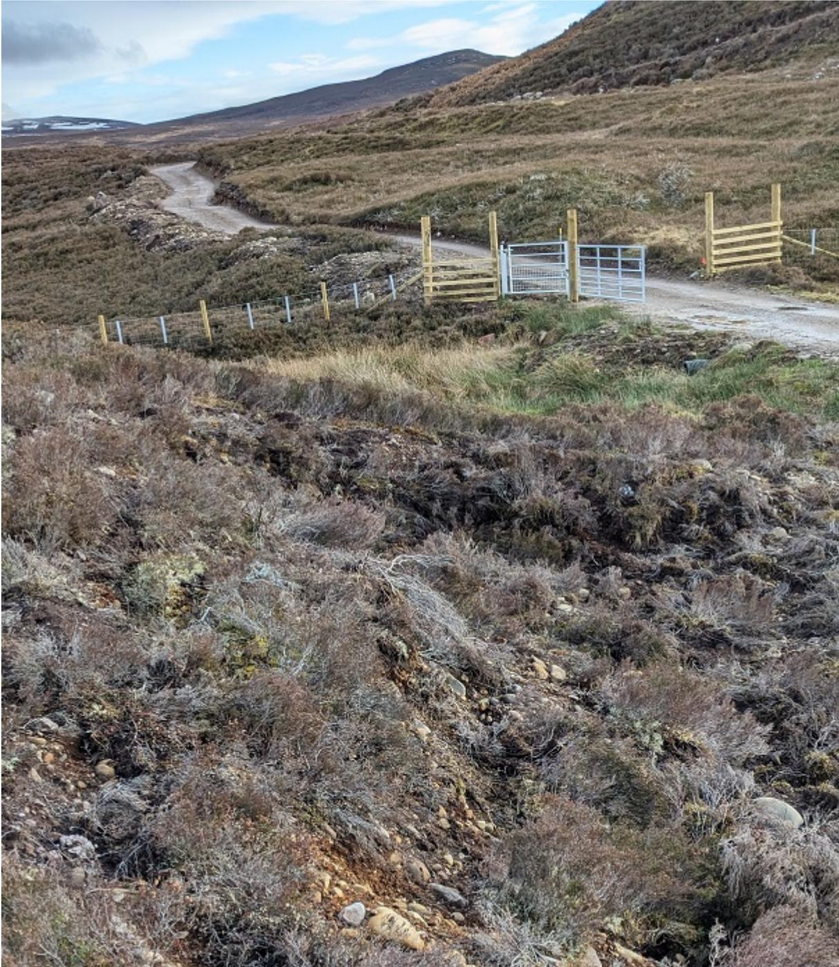
Note not just the borrow pit in the foreground, which has been partially covered up with heather, but the plastic culvert just before the gate and the new bank alongside the road beyond the fence
