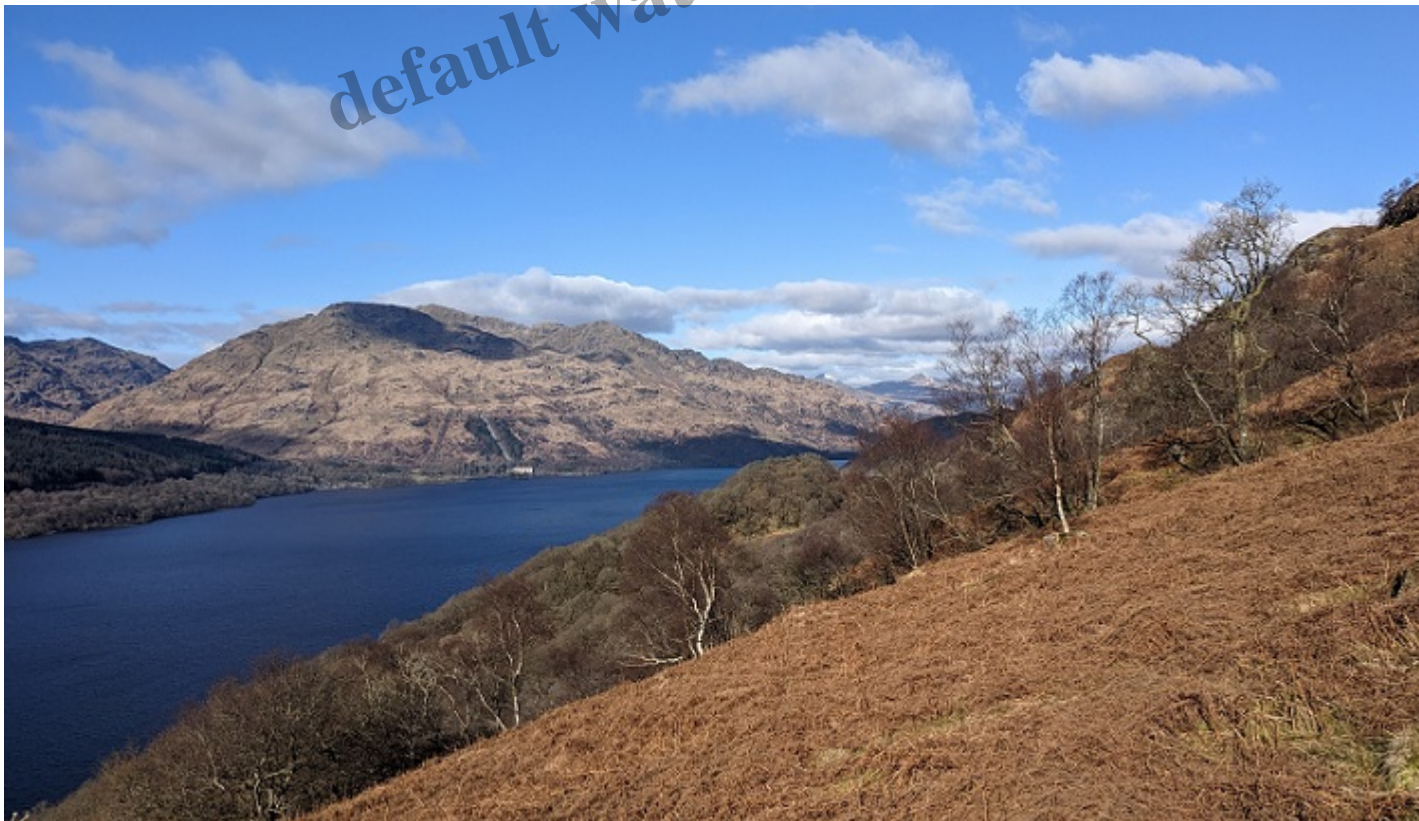
The Loch Sloy power station and feeder pipes above Loch Lomond – if retrofitted it will have a minimal impact on water levels. Photo 2023.
