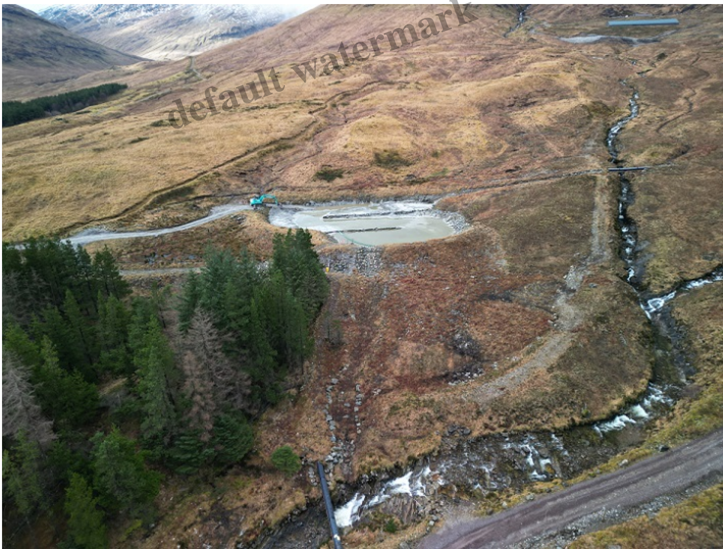
The largest settlement pond with tailings stack 2 and mine shed visible top right, The pipe, centre
