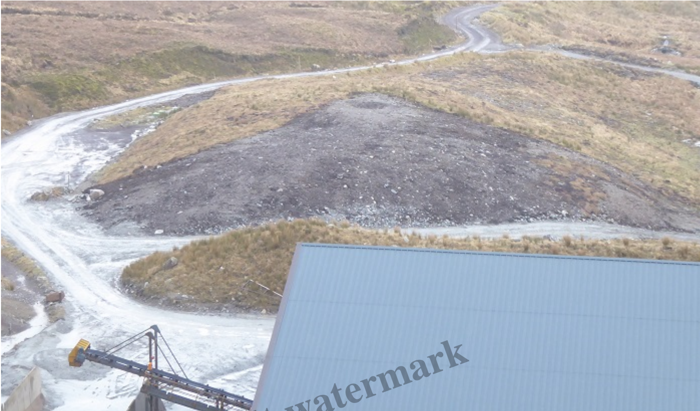
View over roof of production shed showing unrestored area on Stack 1 and the amount of silt on site six months after production ceased and all the winter rain
