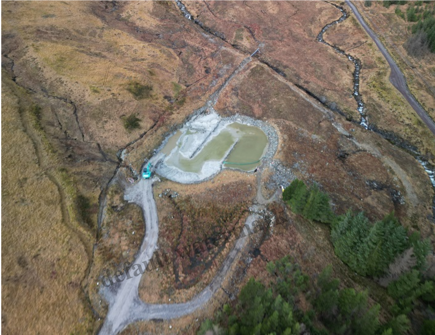
Lower settlement pond still full of sediment six months after the mine ceased to operate. Photo credited to Harry Barnes.
