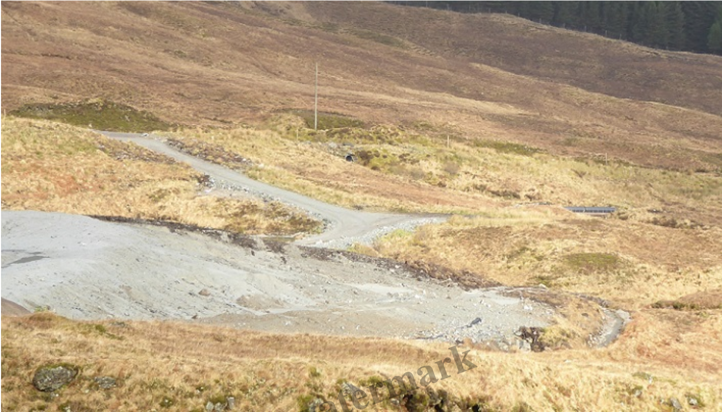
Tailings stack 2 with the drainage ditch designed to catch run-off visible below. The side of the main heap has clearly been eroded by water.
