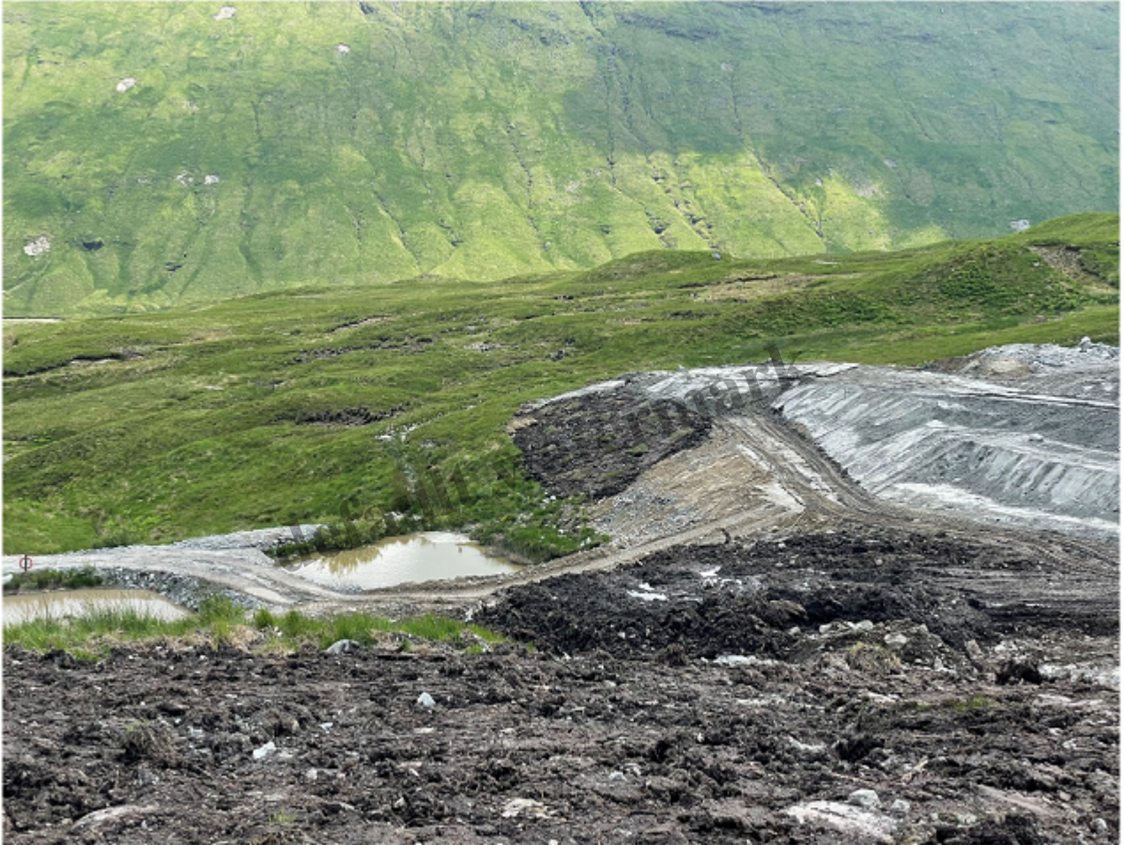
Formation of HEA3 between Stack 1 and Stack 2 continues along with progressive restoration of Stack 2
