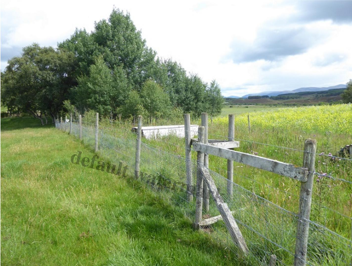
Stock fencing at Ralia with wire mesh. In this example the purpose of the fence is to keep livestock out of a gamebird rearing area, not woodland.
