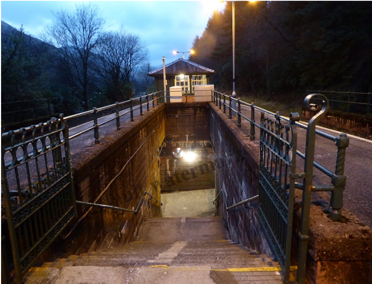
The access to the platform at Arrochar and Tarbet station
