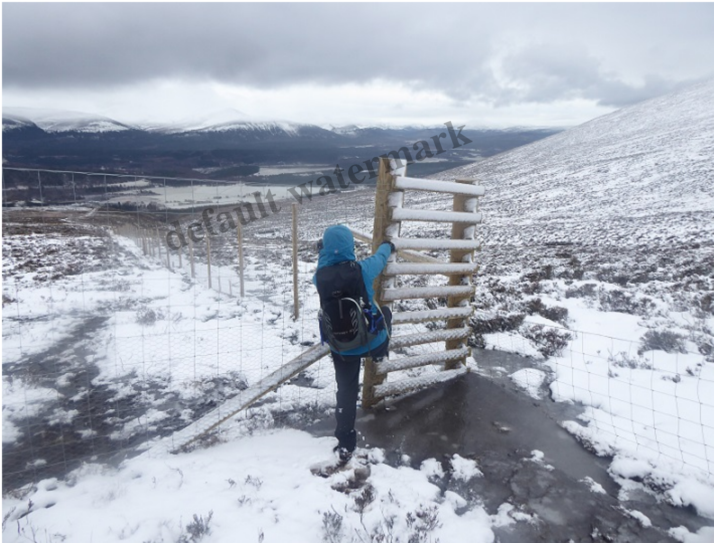
The north west corner of the boundary fence 30th December. Note how the lower horizontal wooden slats are covered in wire mesh making it difficult for feet to get a purchase.
