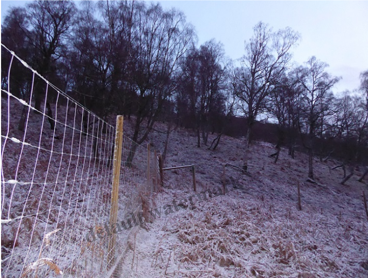
Deer fencing by the gate on the Burma Rd (top photo).
