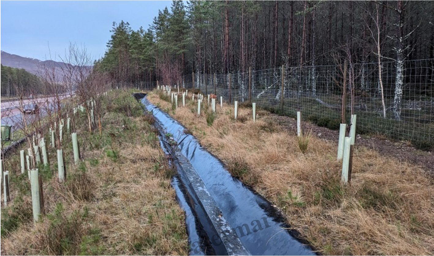
Southbound layby on dualled section of A9 south of Aviemore with lots of polluting plastic and dead, unmarked deer fencing
