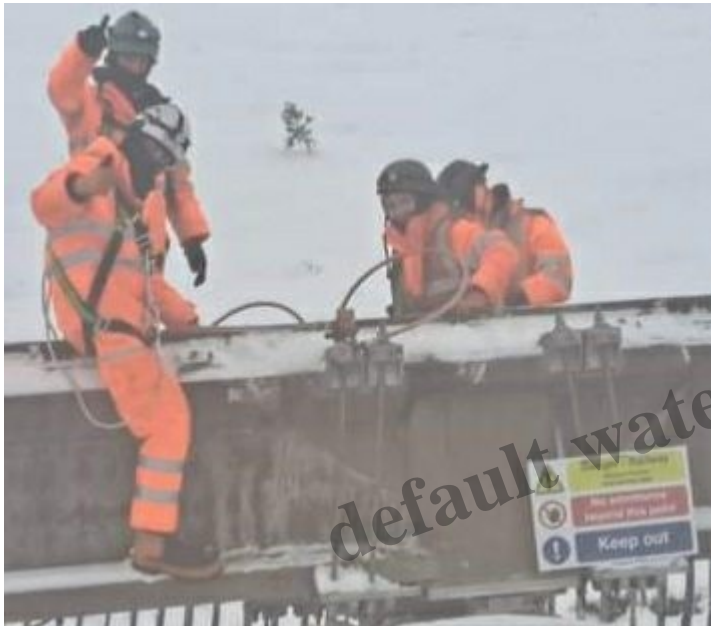
Workmen on the tracks during the w/end of 2/3 December. The metal brackets in the photo are to prevent the scarf joints breaking up.
