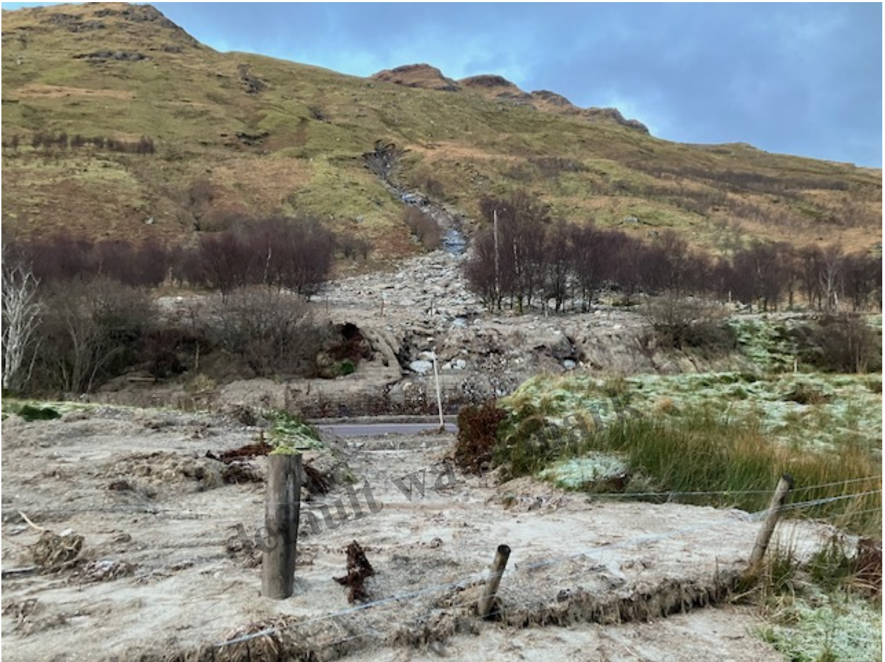
Landslip on the A83, the first below Butterbridge, taken a little further west than the previous one. Photo credit Nick Halls
