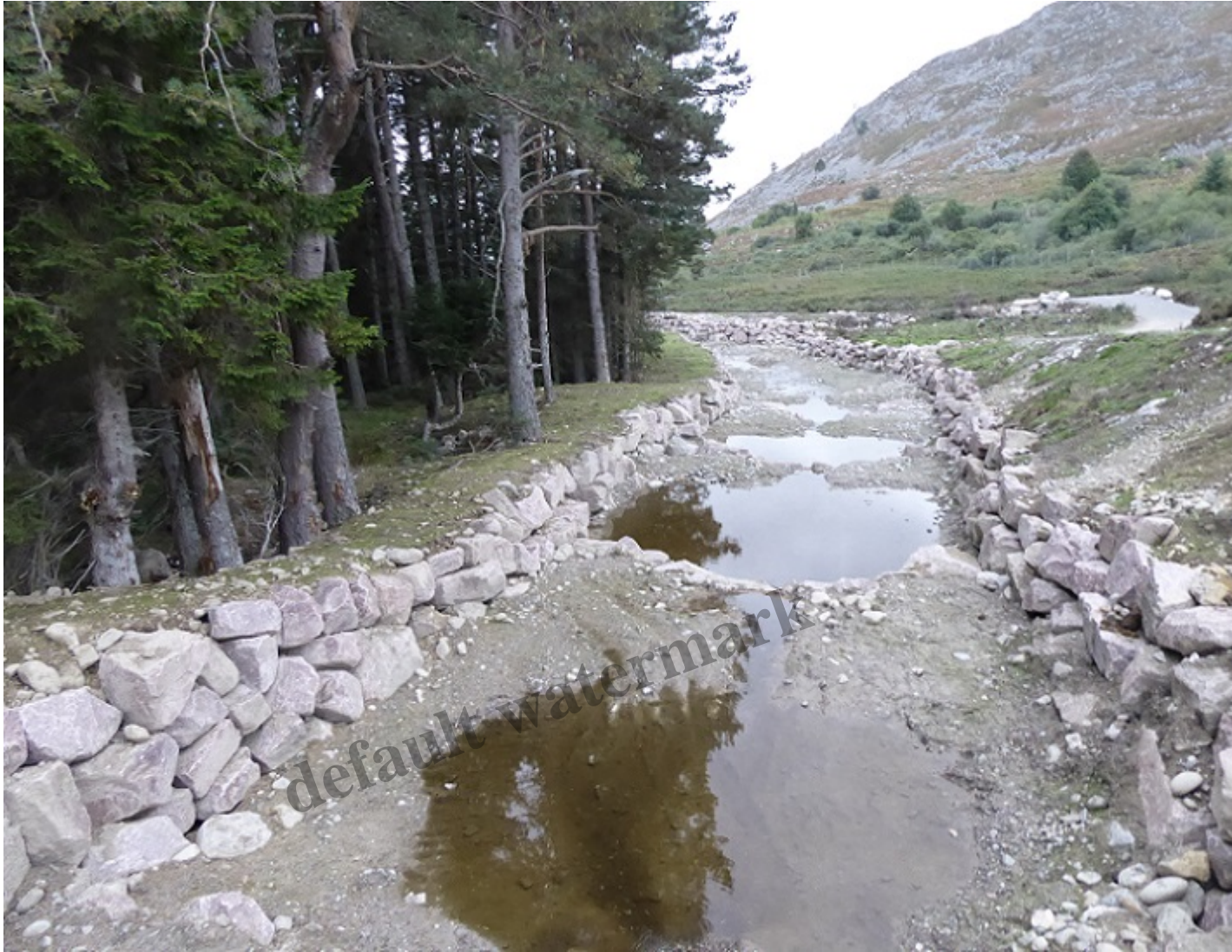
The view downstream from the bridge
