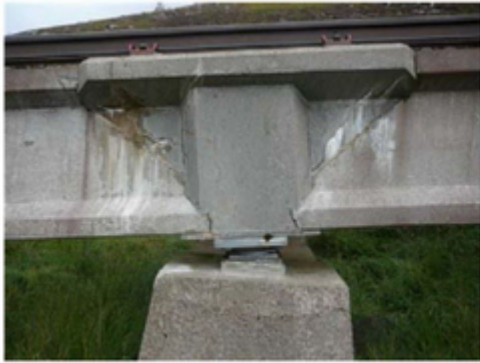
Photo [12] Pier 8, one of the poorer insitu infills. Showing joints opening between Insitu and precast plus cracking within the mass of the Insitu, both inclined and near vertical.
