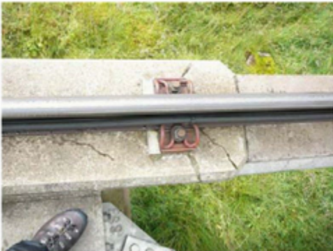
Photo [13] Pier 8 from above.
