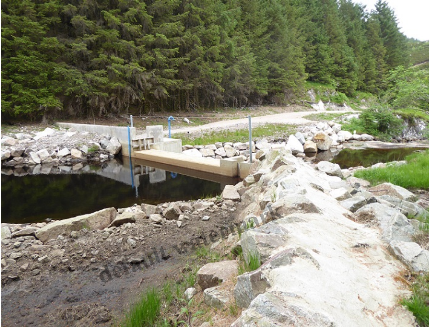
Intake with raised walls to stop the All Bhiorain changing course in flood
