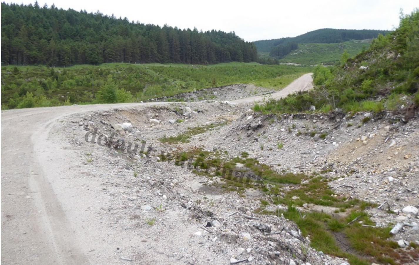
New section of track connecting the power house to the forest road network. Note how the side of the track, just beyond the bend, is washing away.
