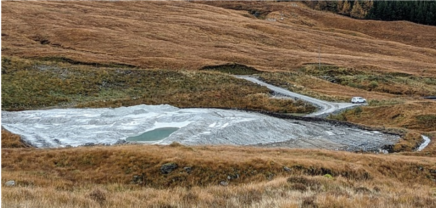
Stack 2 tailings 25th October with artificial drainage channel visible on the right. Note the amount of water sitting on the top surface of the stack and the water erosion channels running down its right hand side.
