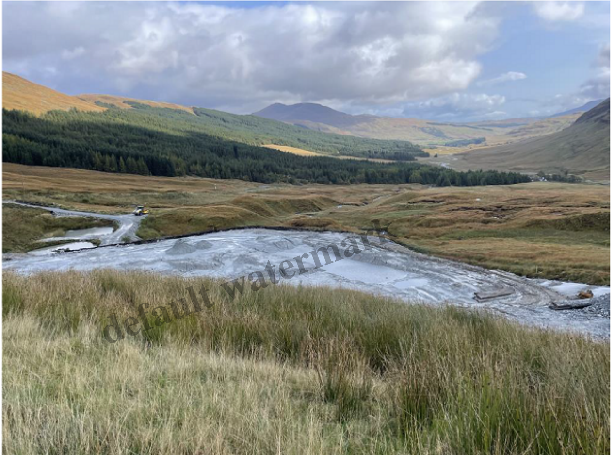
Image 2: Progress on Stack 2 (October 2023)
