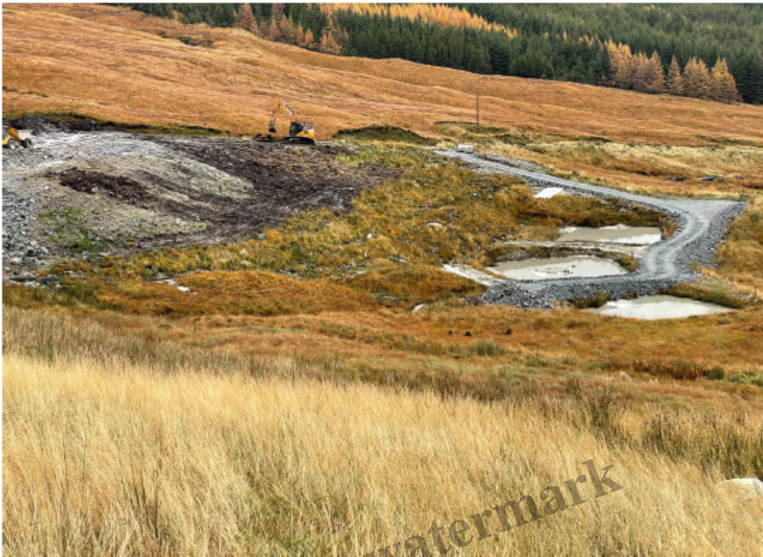
Stack 1 restoration and HEA 2 location, existing ponds to be drained prior to formation of Stack 2
