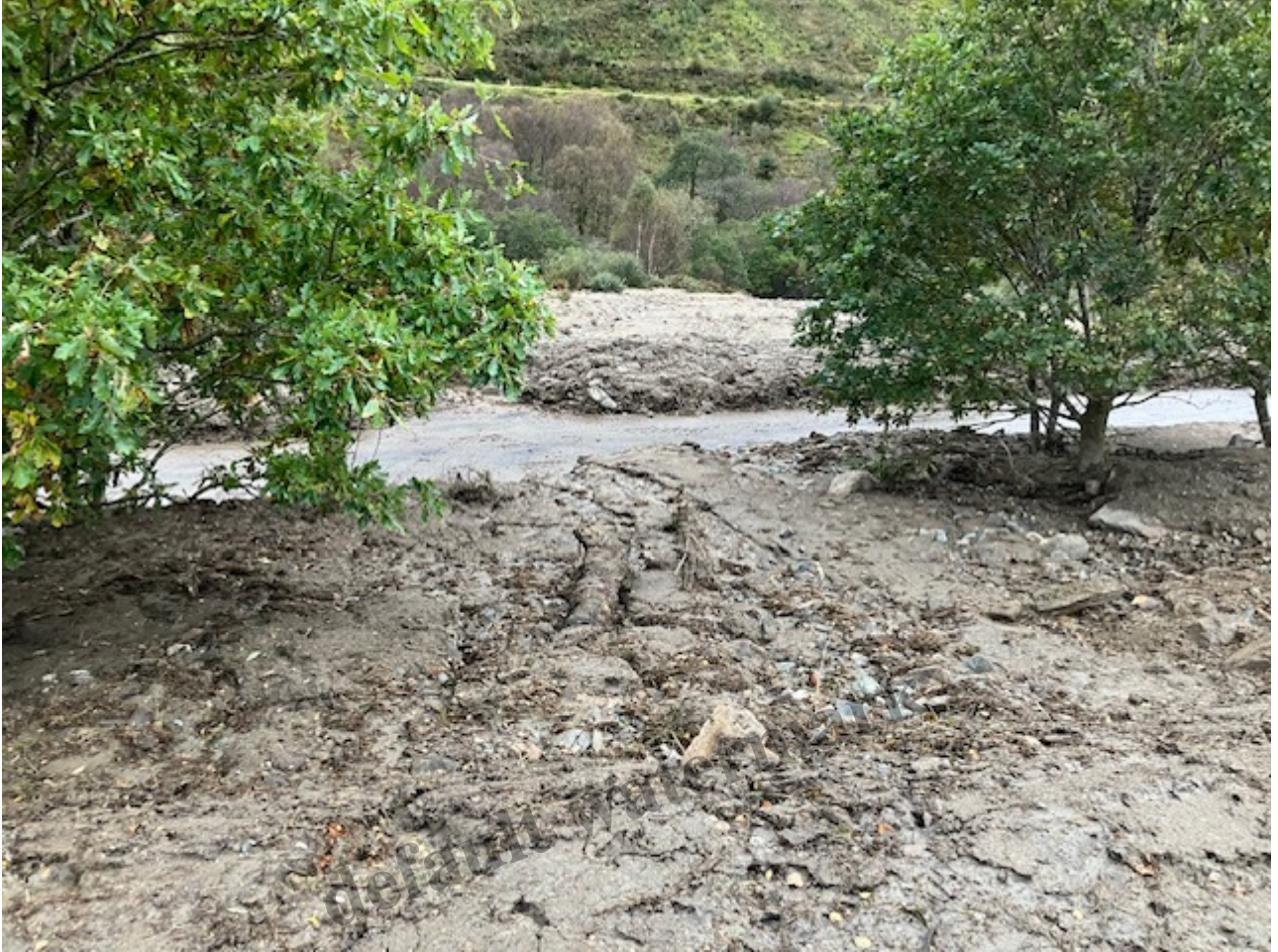
One of the recent landslips that crossed the A83 showing the volume of material and how mature trees can help. Photo credit Nick halls
