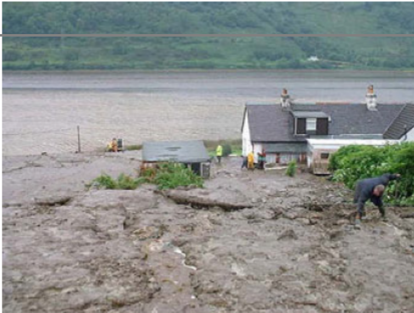
Figure 2.4 – Debris flow above the A83 to the west of Cairndow showing the effects on a roadside cottage and the trunk road immediately downslope from the cottage.
