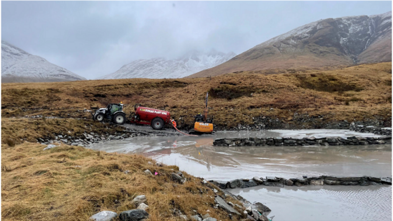
Pond – removal of accumulated silts/ sludge
