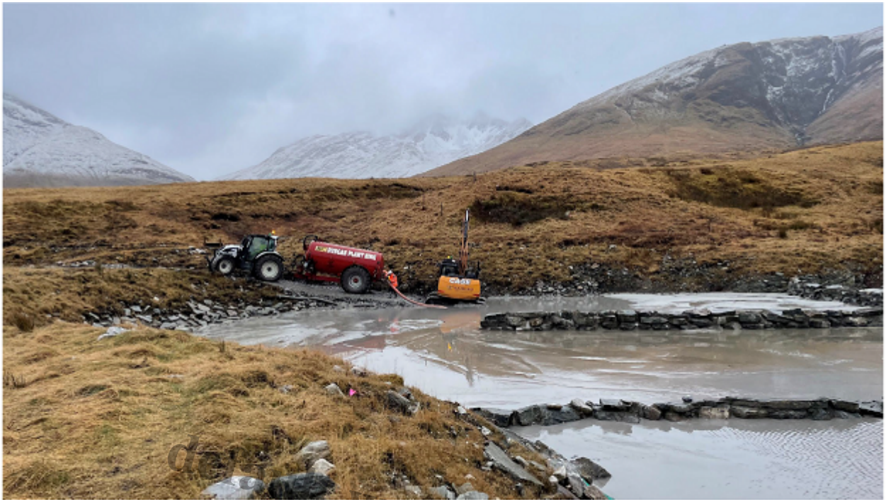
Pond – removal of accumulated silts/ sludge
