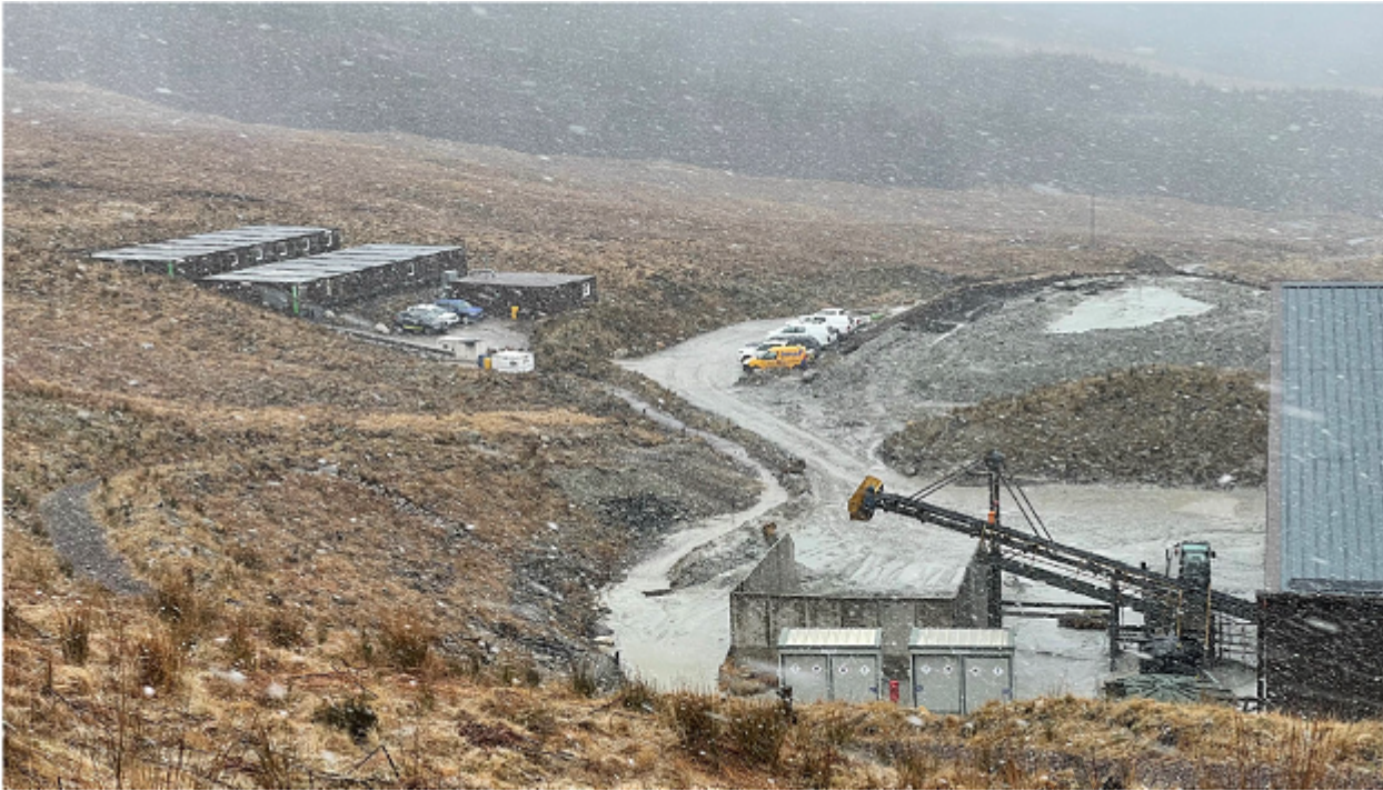
Stack 1 restoration progress – overview from Mine site platform
