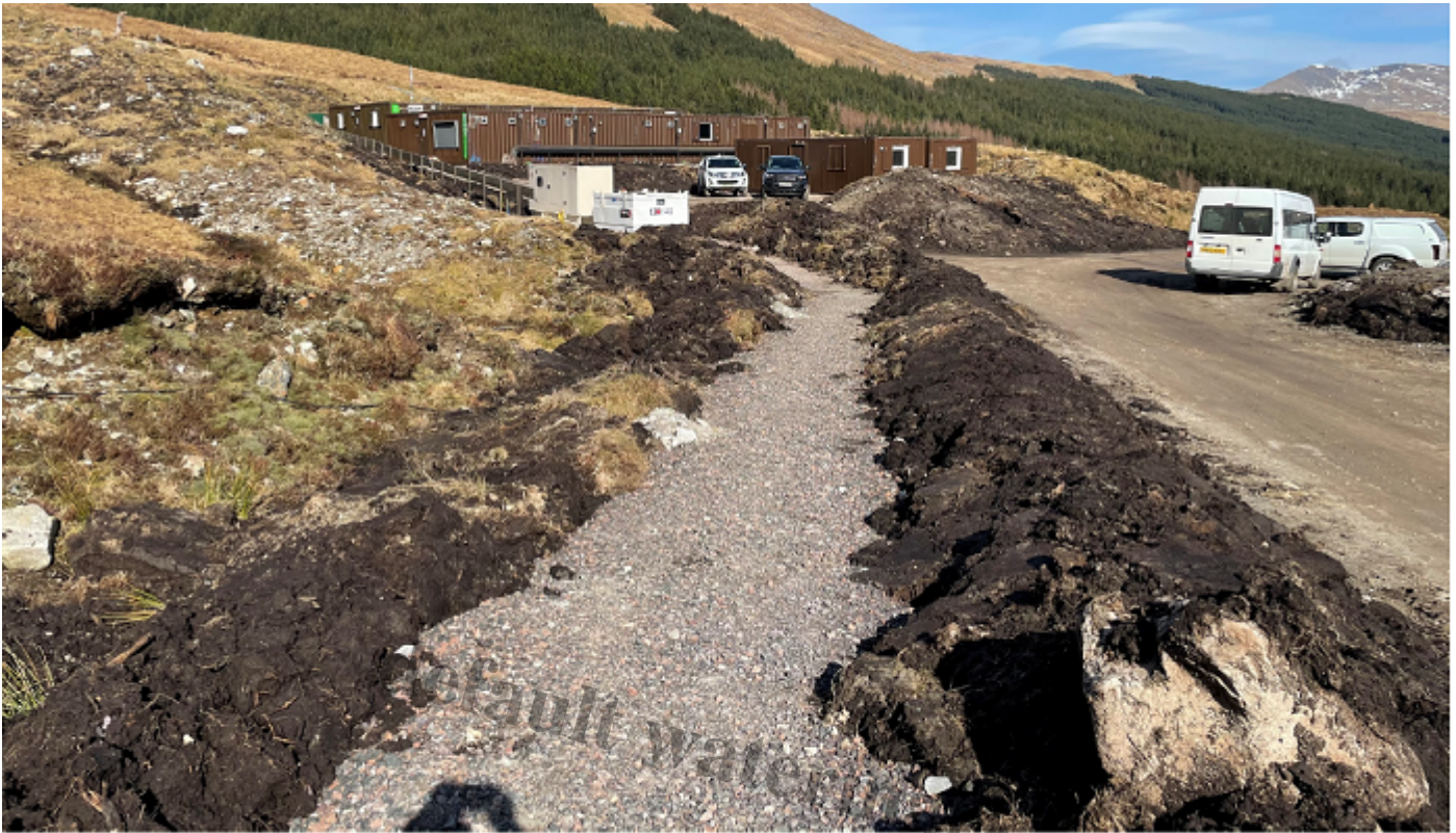
Walkway extends to the contractor's temporary compound, clarification of permanent / temporary nature of walkway at this location?
