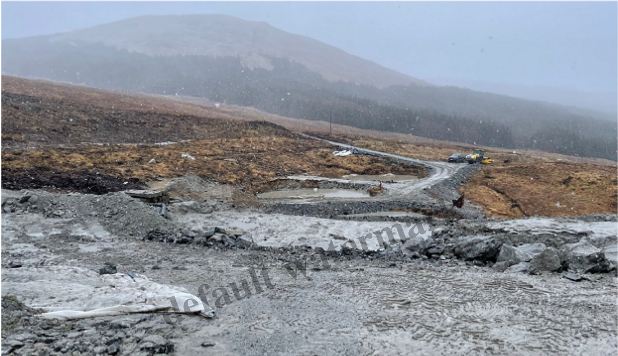
Stack 2 – Initial deposit of tailings as per KP Technical Note/ phased approach
