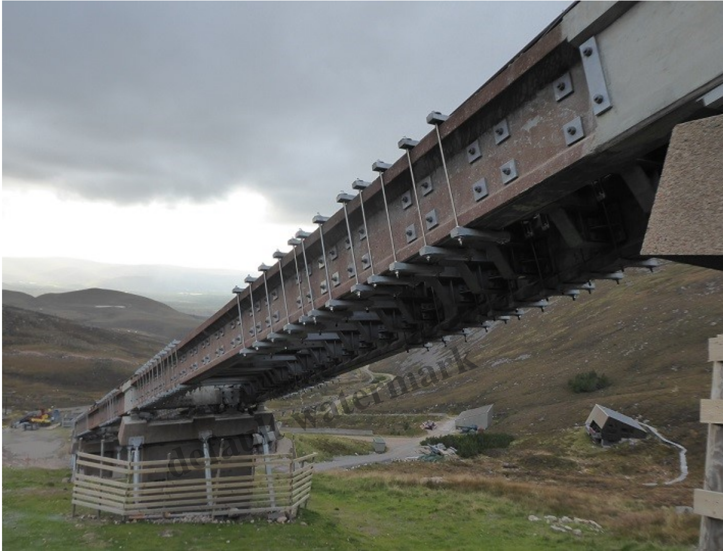
Photo showing the extensive use of metal reinforcing brackets by the mid-station
