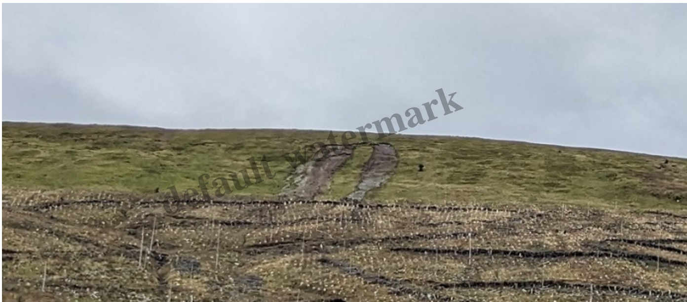
Parallel landslips above destructive forest harvesting in Glen Lean, just outside the National Park boundary
