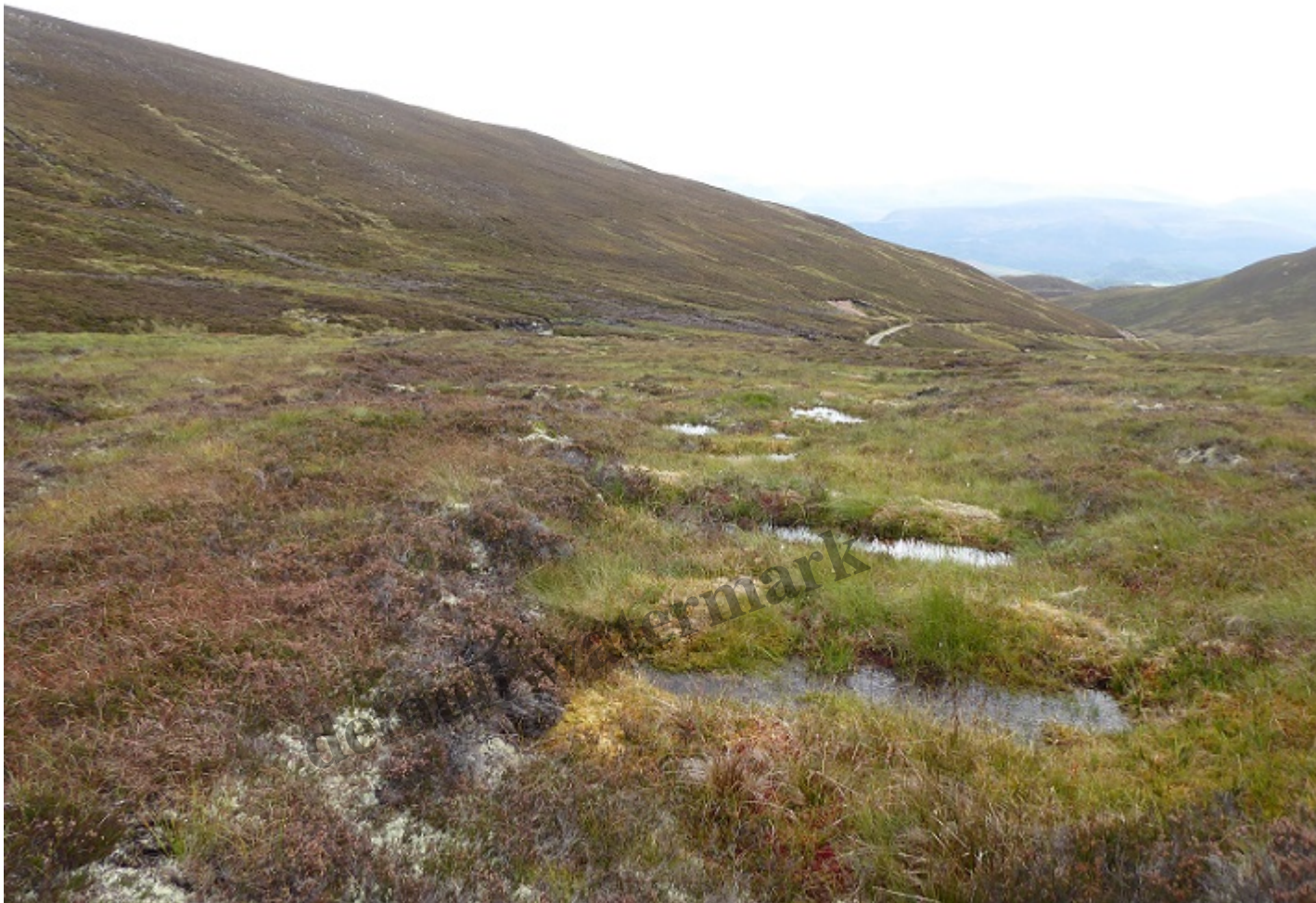
Blocked drain from above with Burma Rd and borrow pit below. Mounding is just visible running up hillside left of centre
