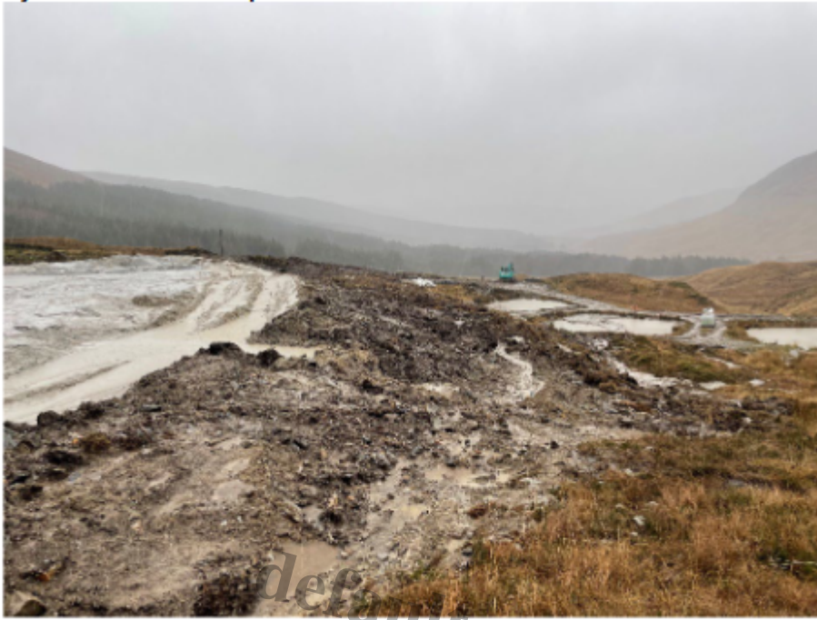
Stack 1 formation and restoration, series 3 old lagoons below Stack 1
