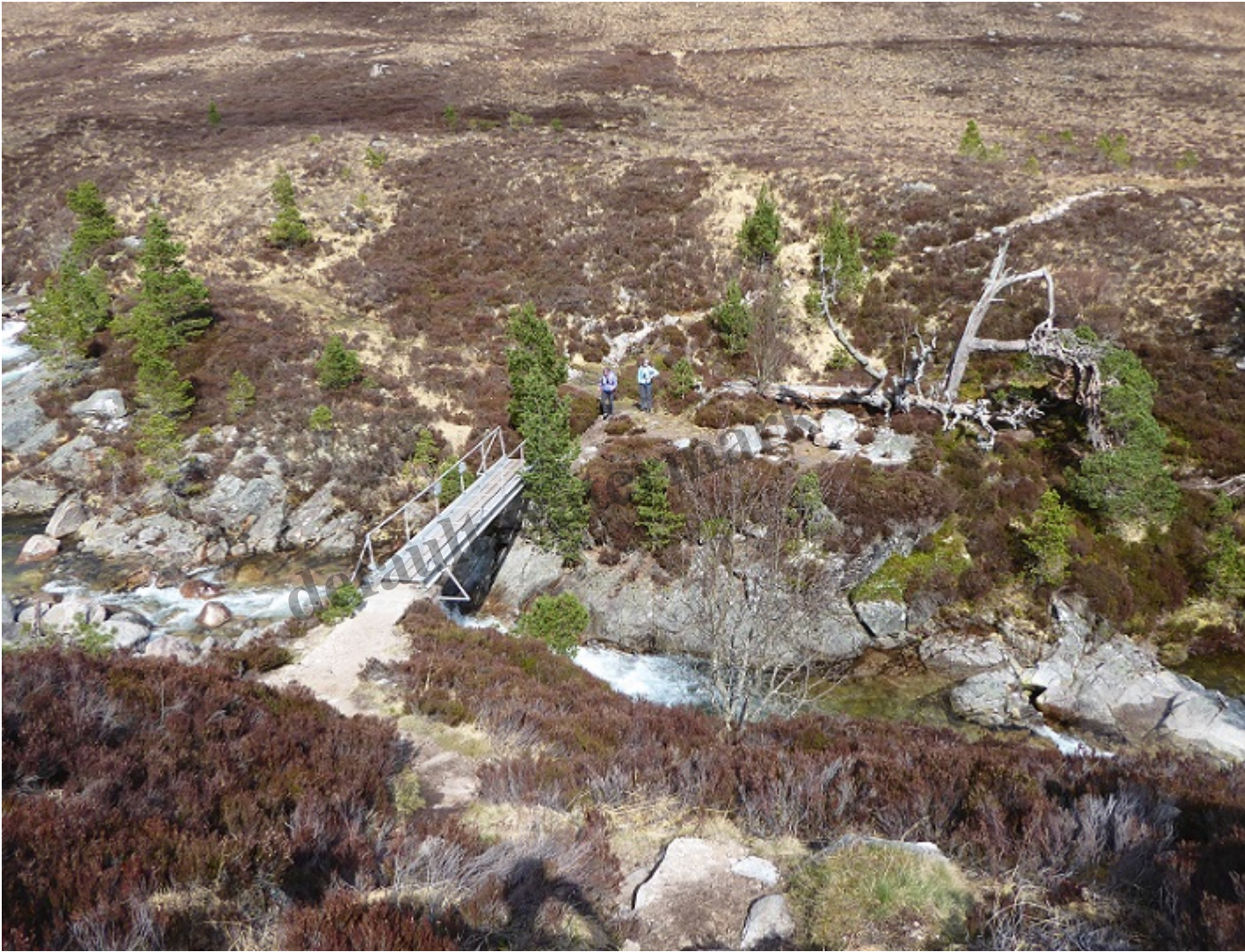
The bridge over the Luibeg burn 2018 showing peat bog and naturally regenerating Caledonian pine forest. The proposed mast would be on the high ground behind the viewer.
