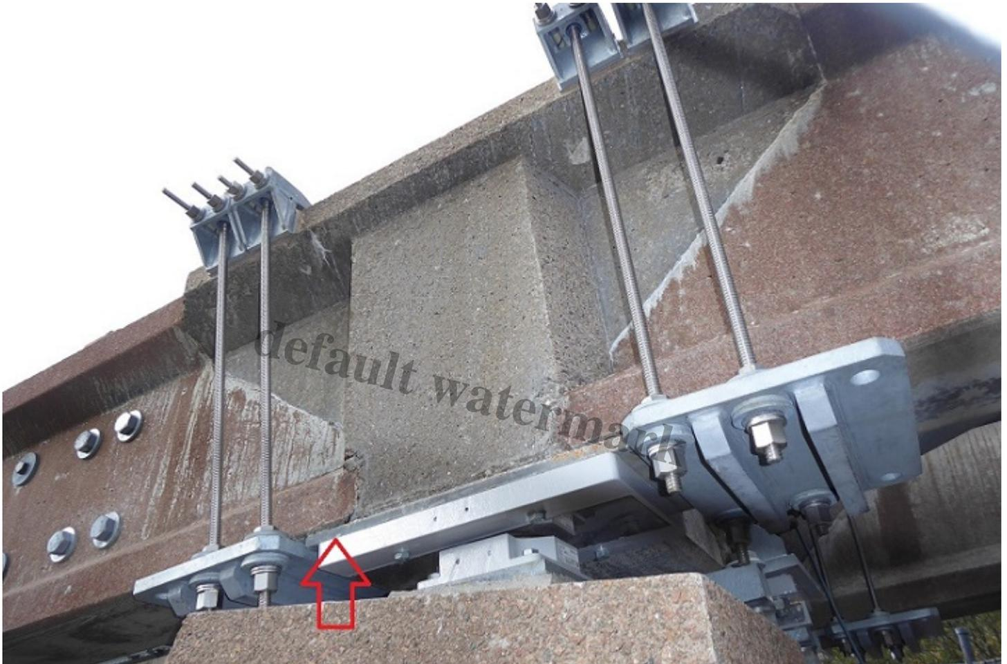
The red arrow shows how the original supporting plate has been retained although the bearing and support below it have been replaced.
