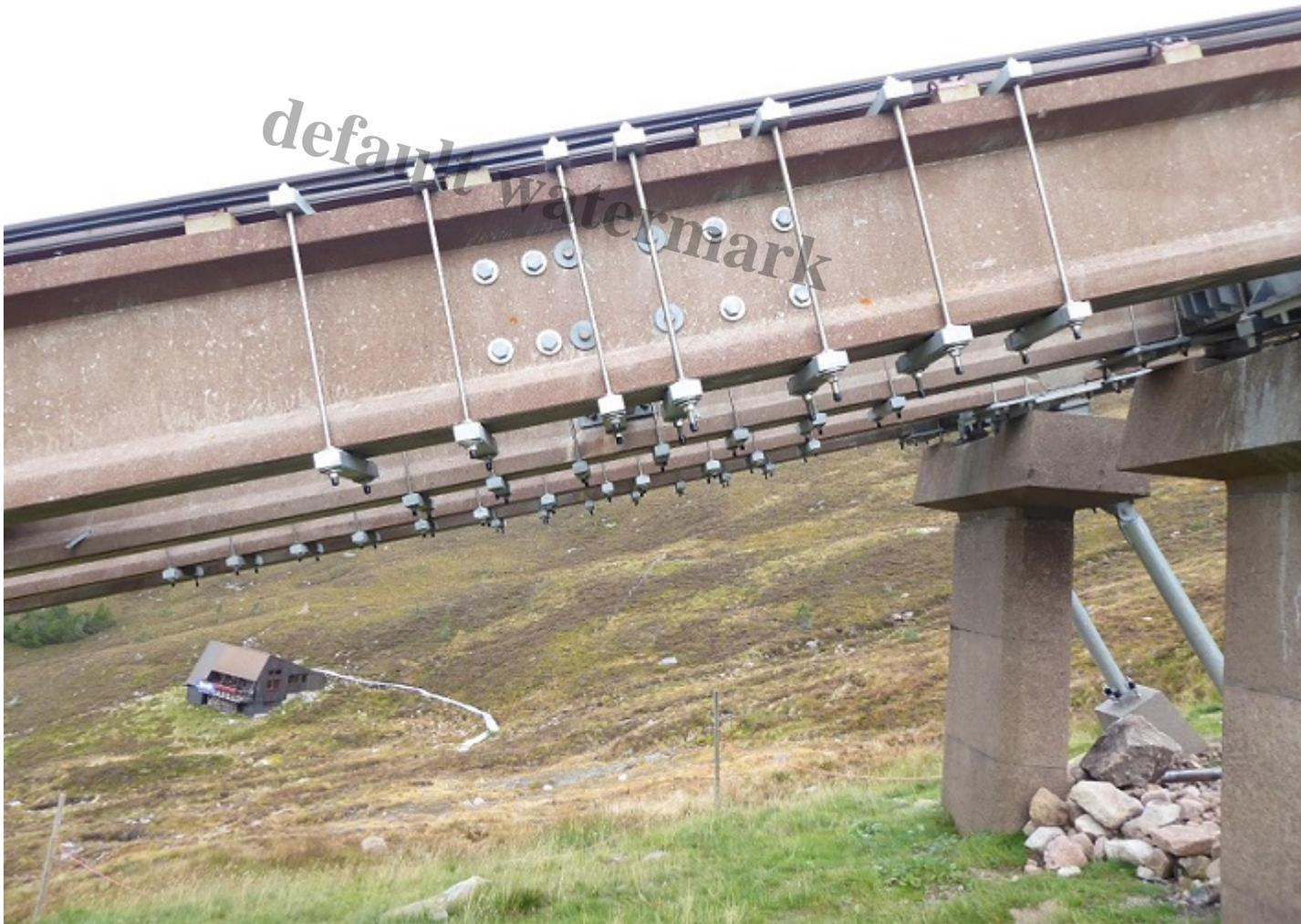
Photo showing how different additional brackets have been placed on each beam, in addition to the pairs around the scarf joints, and how the number of these brackets vary.
