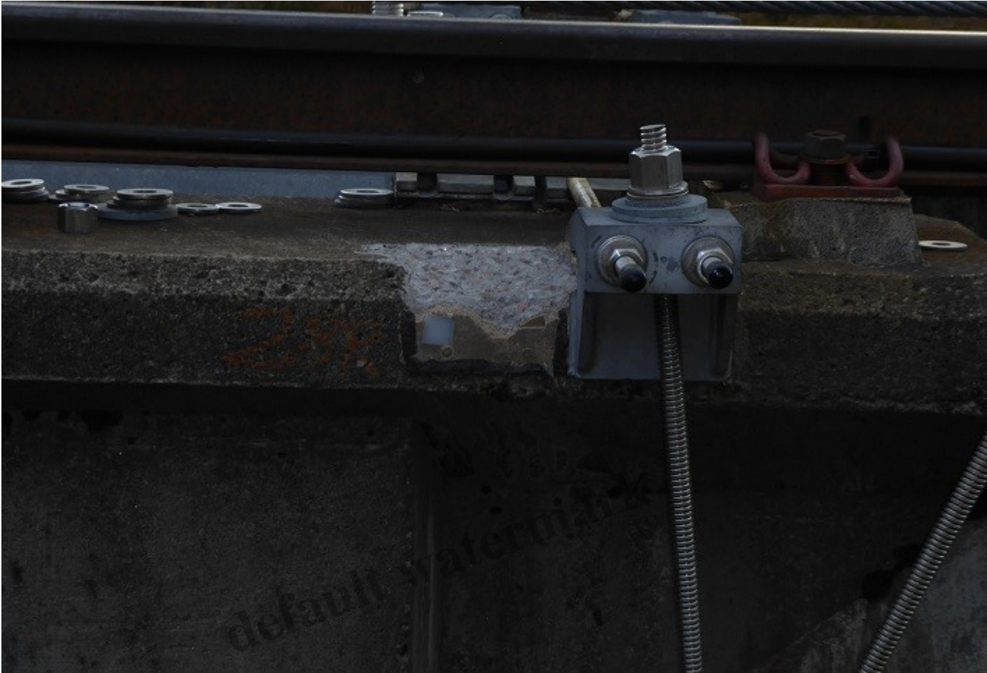
Close up – note the layer of grout on the outside face of the broken concrete
