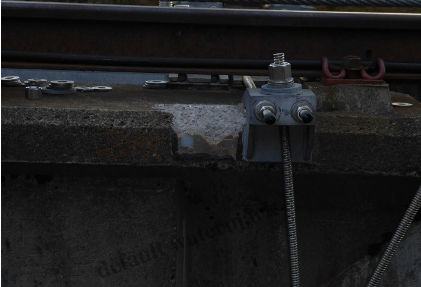
Close up – note the layer of grout on the outside face of the broken concrete
