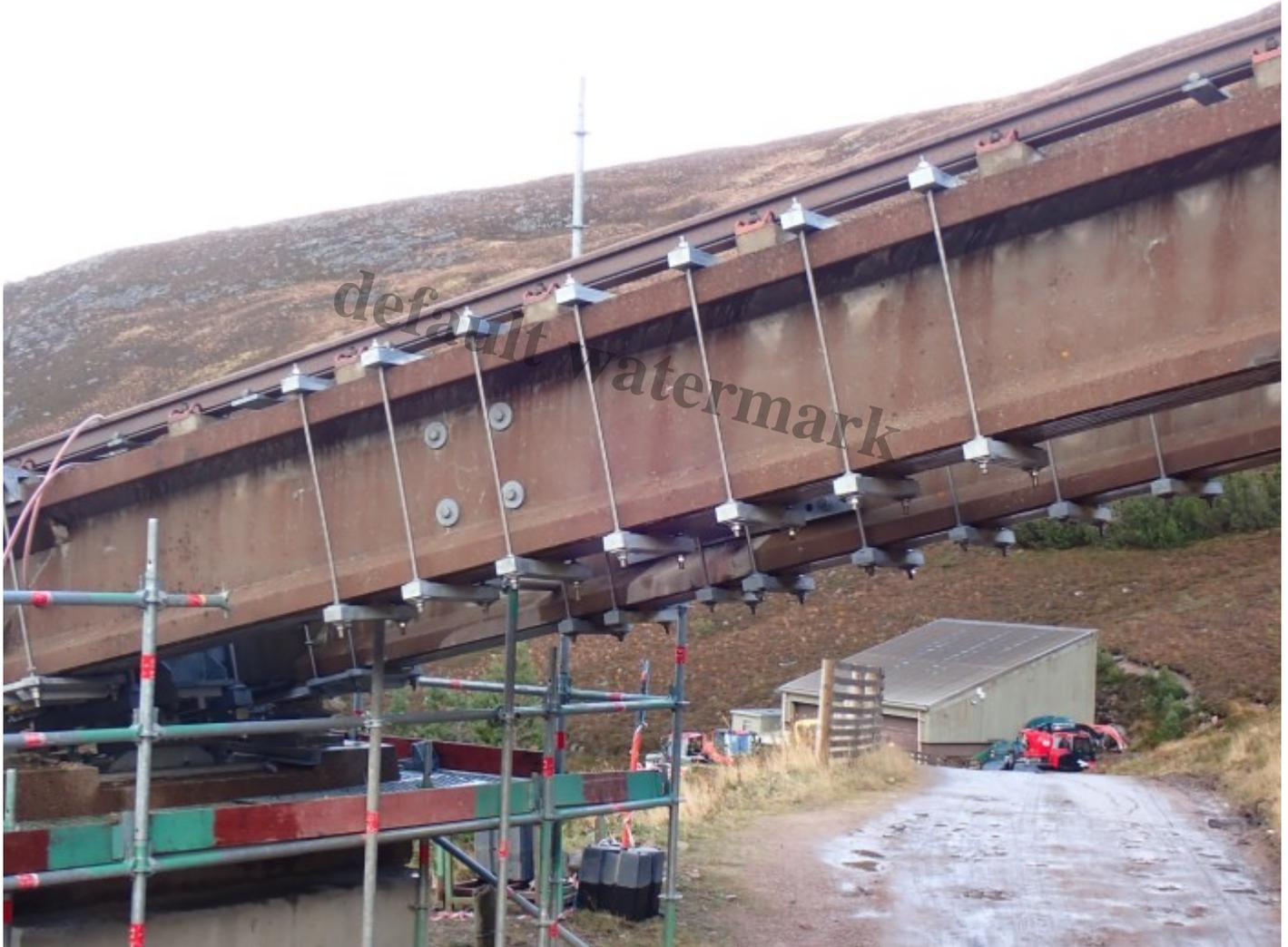
Photo courtesy of PW reader showing reinforcement of an I-beam below the Shieling.
