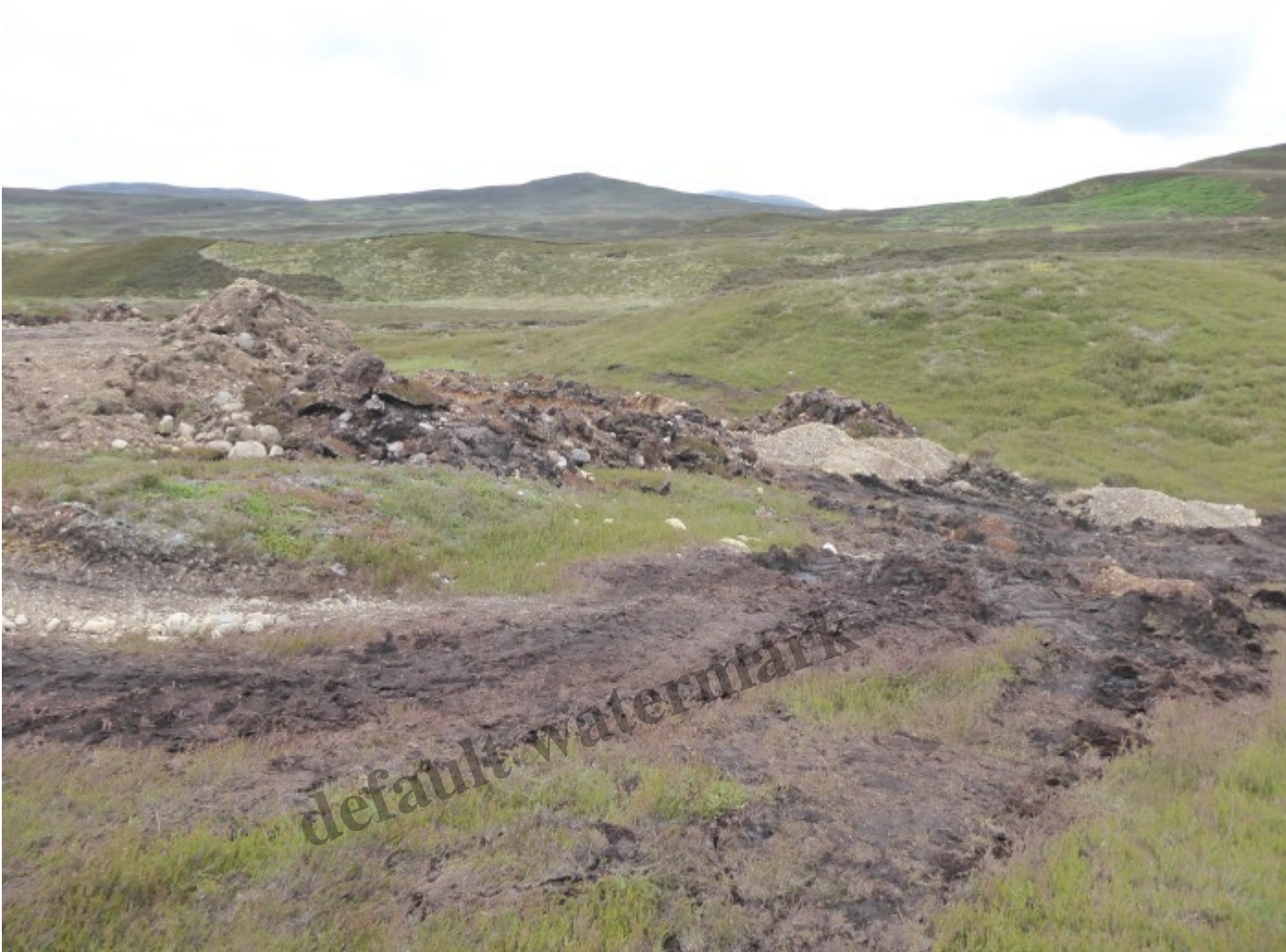
The quarry at the end of the peat road seen from above
