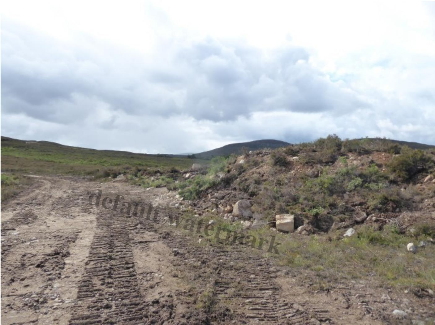
Another restored borrow pit albeit by a section of the road which has been widened excessively
