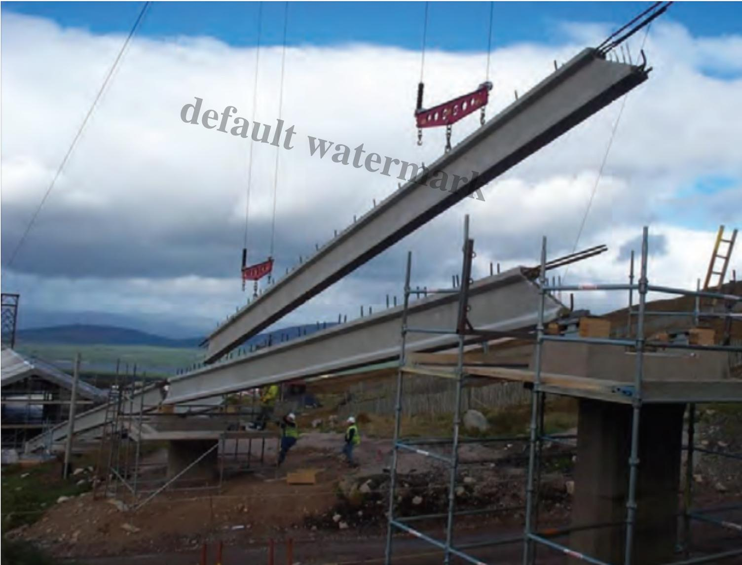
Note the concrete beam is being lowered into place using the aerial cableway.
